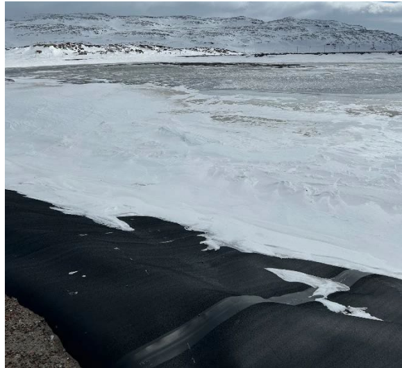
Figure 2: Kugaaruk Sewage Lagoon Liner Bubble, April 2024
