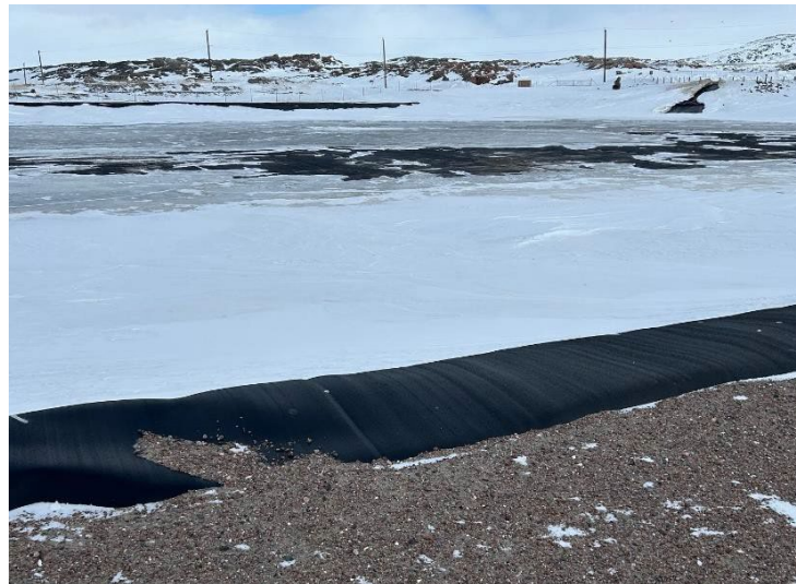
Figure 3: Kugaaruk Sewage Lagoon Liner Bubble, April 2024
