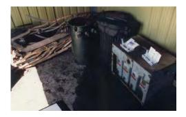
PCB capacitors that are thrown into bins with other PCB waste will have to be separated from such waste prior to being removed from the site for disposal. The exercise of dividing PCB waste into compatible types is necessary since the disposal costs/kg vary considerably from one waste type to another. Also, depending on the type of PCB waste, they may be treated at a number of different transfer stations or destruction facilities.
