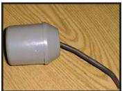
Sump pump float containing mercury.
