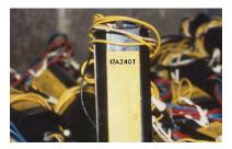
Sometimes ballast labels are difficult or impossible to read or have been removed altogether. It should be assumed that they are PCB type if they appear to be of the same vintage as the other ballasts in the lights or based on the age of the building, that is, older than 1980.
