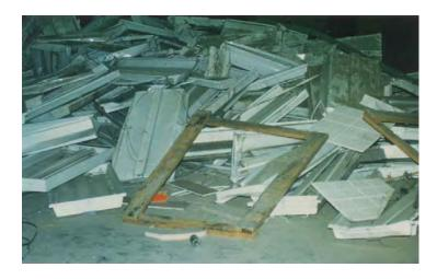
An area designated for storing ballasts removed from fixtures should be identified prior to a job and all workers should be required to follow proper handling procedures. The following is a summary of the procedures that have been developed and implemented by several groups for the removal and storage of fluorescent light ballasts containing PCB's.
