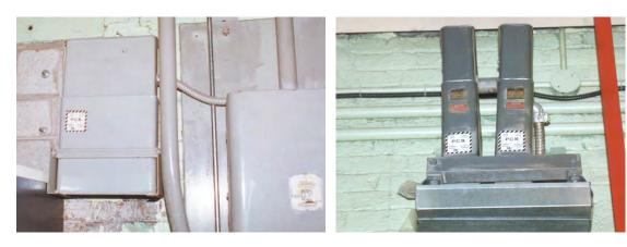
The large OR stickers would be placed on transformers and the smaller ones would be used for labelling capacitors.
