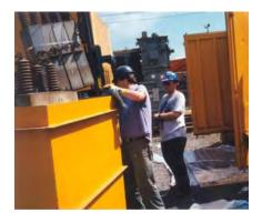
If a client does not mind if the container in which the capacitors are stored is also removed from site to the disposal facility, capacitors may be loaded on trucks in sizable steel boxes. However, the costs for disposal are based on the weight of the capacitors and the container. The large heavy-gauge steel containers will contribute to a significant increase in disposal costs.
