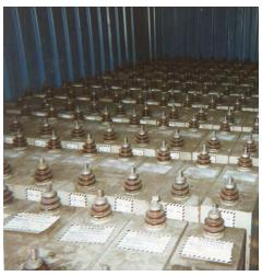
In these cases, when the capacitors are to be removed from site for disposal, they have to be removed one at a time, placed on pallets and banded before loading on the truck. This adds significant costs to the site service charges.
