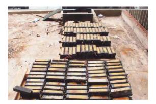
When working indoors, many contractors will place ballasts in the same boxes the non-PCB ballasts came in. This practice just adds to the work when ballasts are later removed, otherwise the boxes add unnecessary weight that will be reflected in higher disposal costs.
