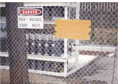
However, there are also PCB-containing capacitors that are cylindrical in shape.
