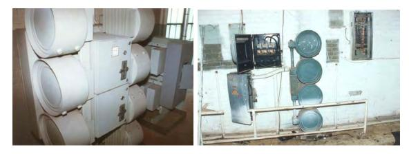
The federal government has kept inventory records of in-service PCB capacitors and askarel transformers and has requested that PCB owners label this equipment with "OR" serialized stickers.
