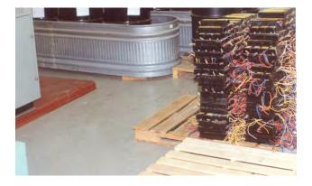
Although it was a common practice to break down ballasts into their component parts on site, this activity is now accomplished at the various transfer stations. The copper coils and capacitor inside ballasts is insulated with asphalt-silica mixture (ASM).
