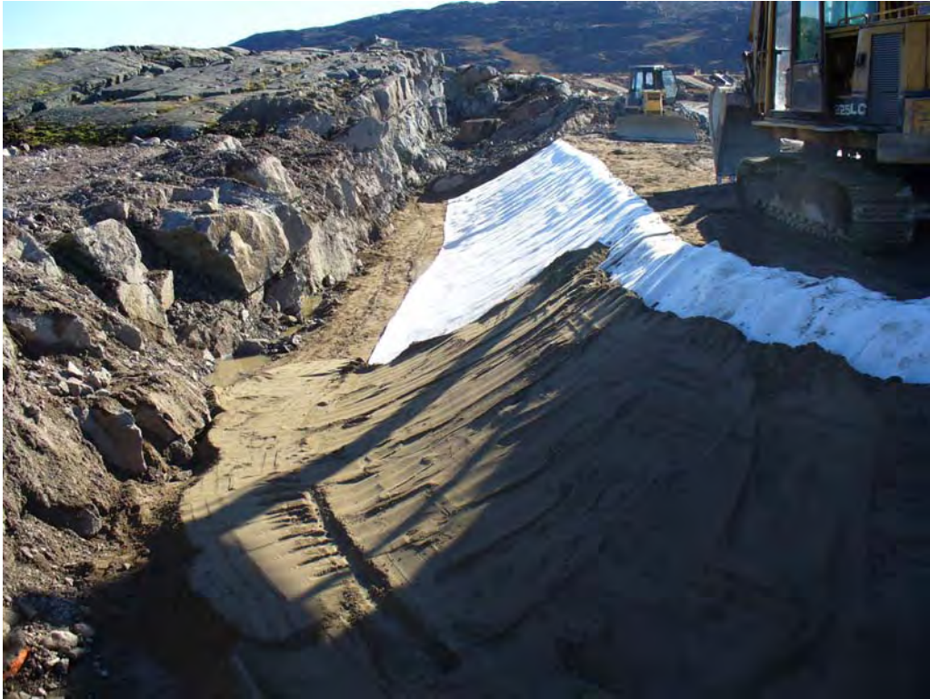
Photograph 5: Placement and backfilling of sand fill atop liner.
