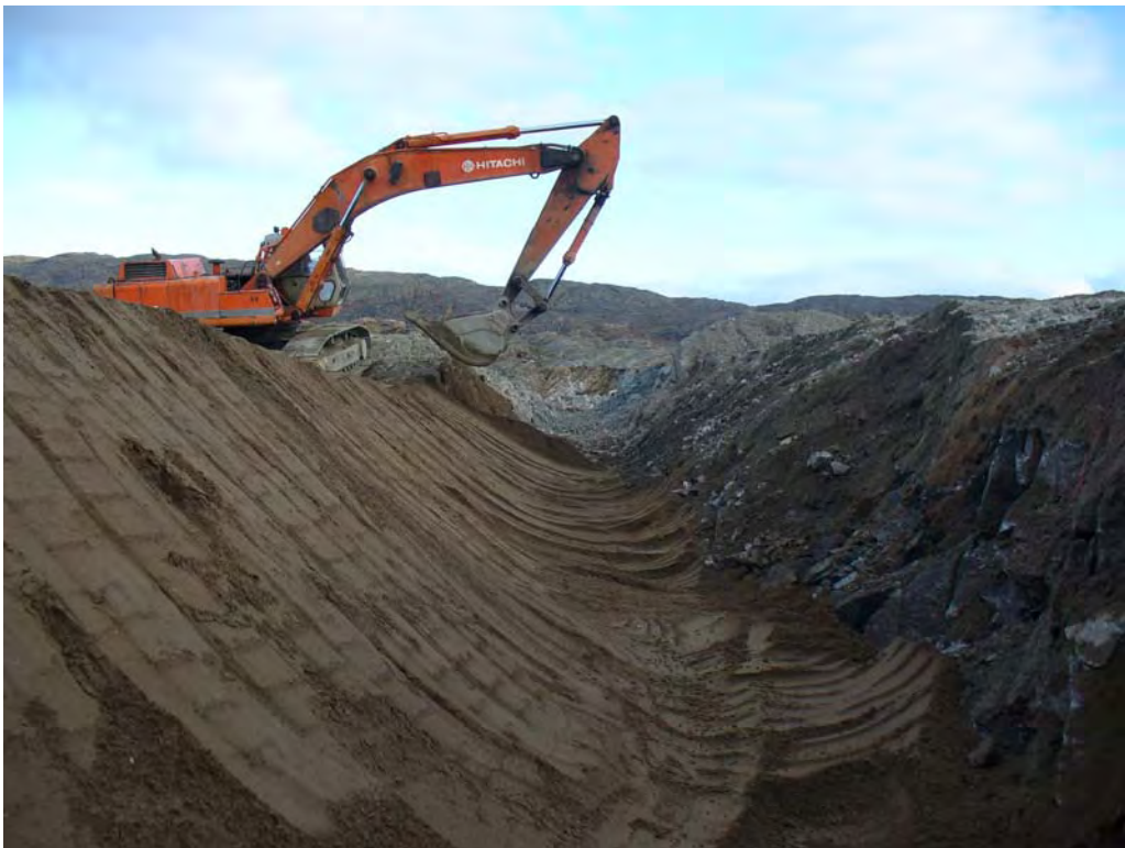
Photograph 4: Excavator placing sand material along trench bottom and slopes.
