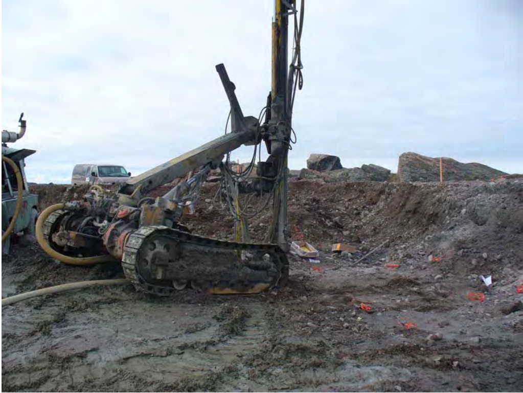
Photograph 1: Track mounted air rotary rig completing blasting holes.
