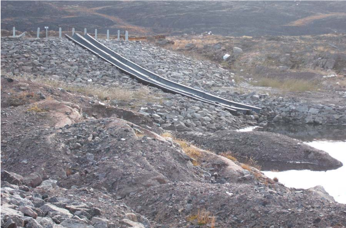
Photograph 3: Southeast slope of lagoon with rip rap blanket and half culverts for unloading effluent from waste trucks into the pond.
