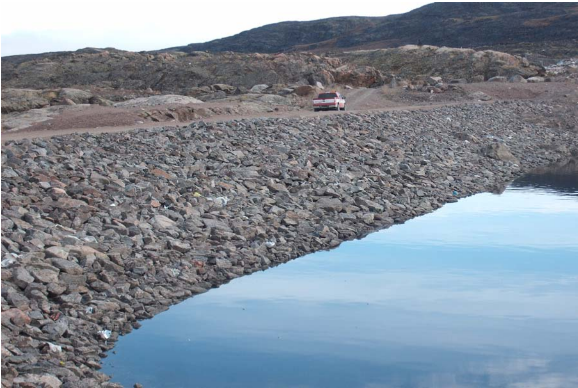
Photograph 10: A portion of northeast berm with rip rap blanket overlying a native rock outcrop.
