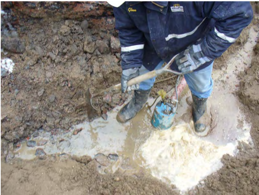
Photograph 6: Groundwater ingress along eastern segment of cut-off trench.
