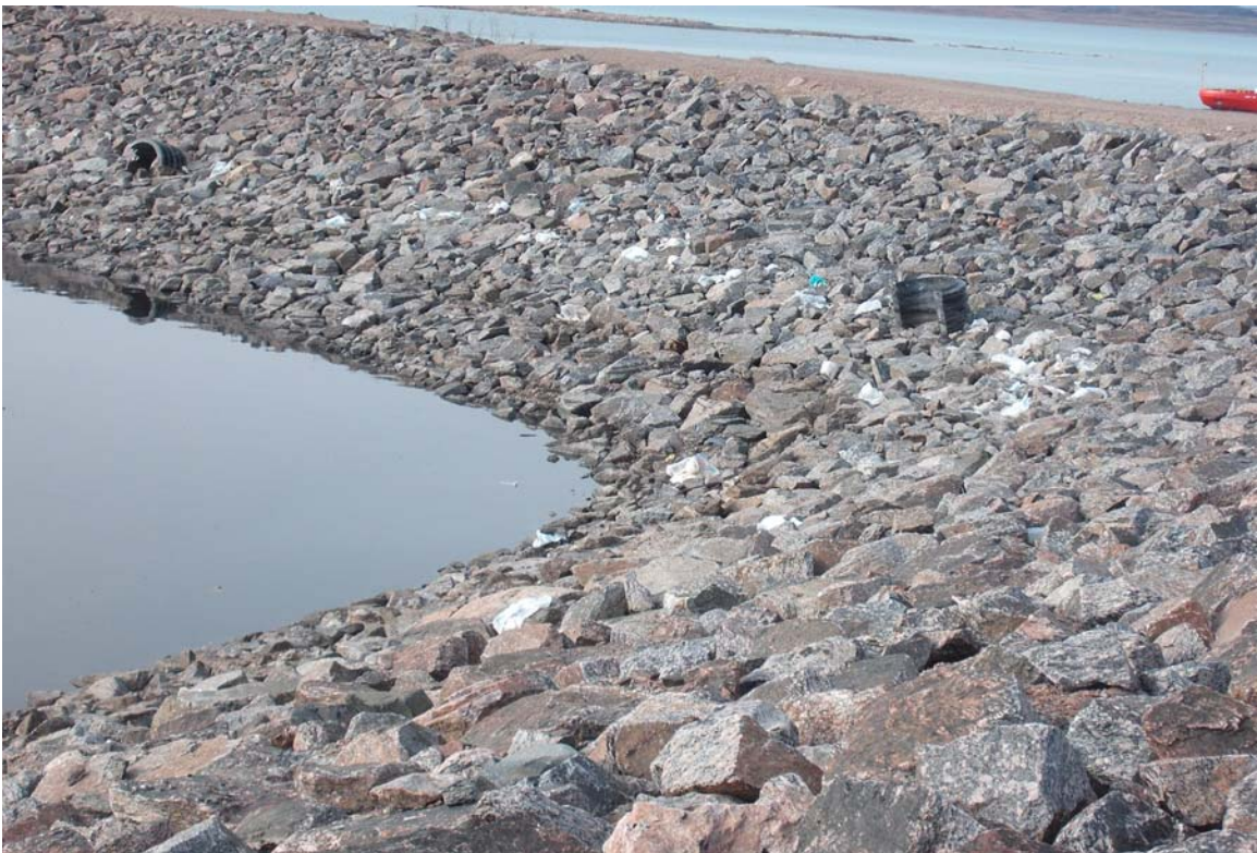
Photograph 2: Northwest berm of dam. Maximum effluent level represented as a broken line of white litter.
