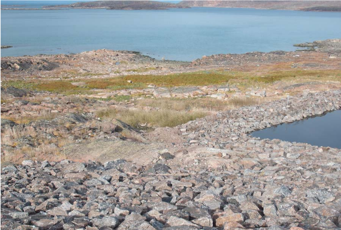
Photograph 17: Terrain downstream from lower pond. Green grass shows area where effluent is seeping below lower pond embankment.
