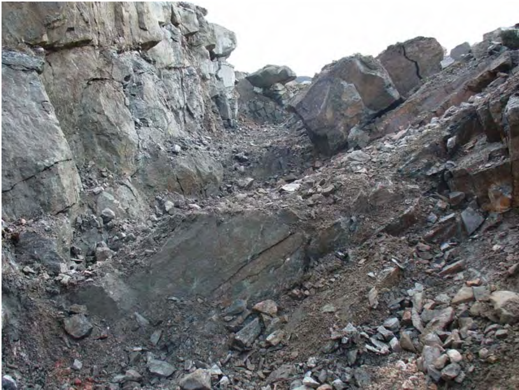
Photograph 2: Eastern segment of cut-off trench excavated in competent and jointed bedrock.
