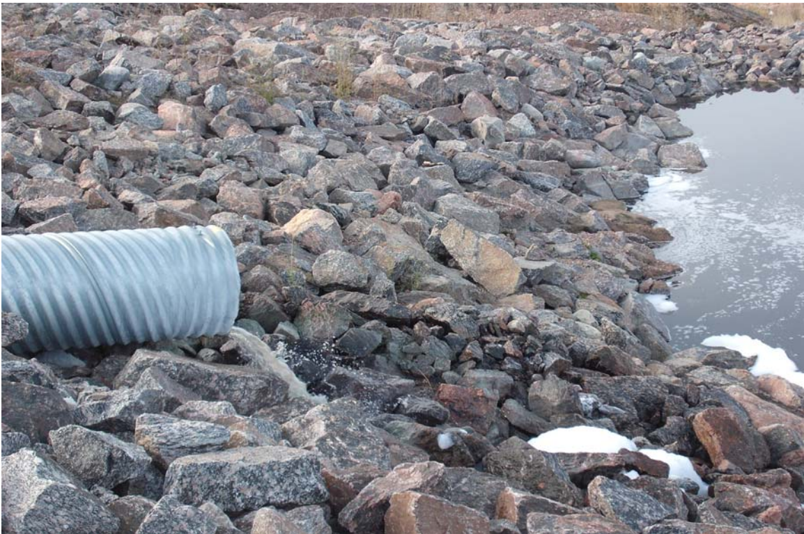
Photograph 12: Close up view of corrugated outfall pipe at external slope of northwest berm.
