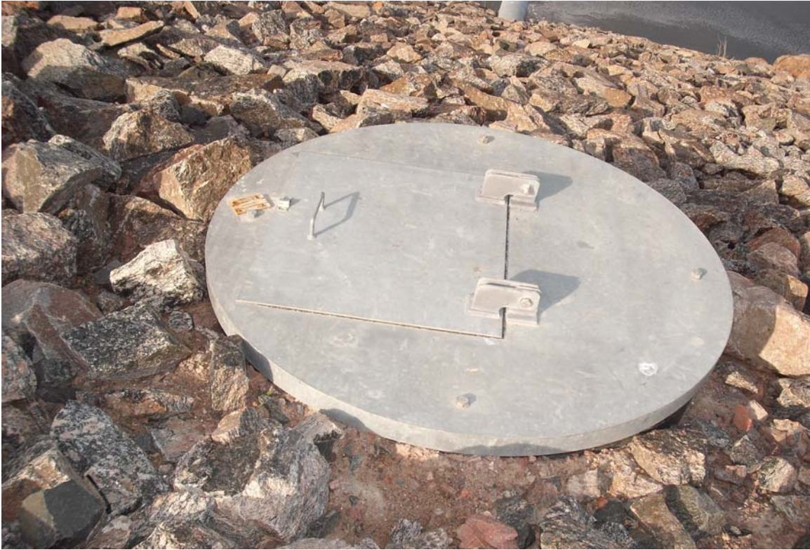
Photograph 13: Manhole lid with no hasp or padlock.
