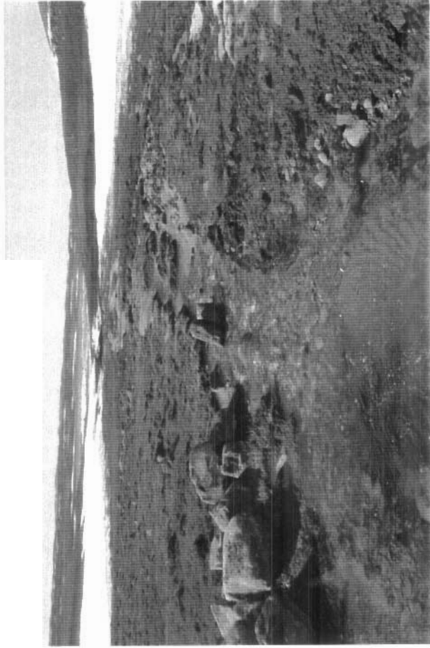
Plate 5 Km 18 Culvert, 30 June 2002. Resting pool on downstream end of culvert during high flow. Note: flowing water allowing fish passage to and from the Alliarusiq River.
