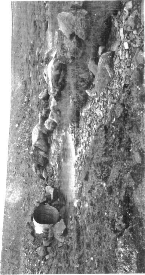
Plate 1 Km 18 Culvert, 7 August 2002. Resting pool on downstream end of culvert. Note: the deflecting dyke situated outside of wetted channel and very little flow through the culvert and in downstream channel.
