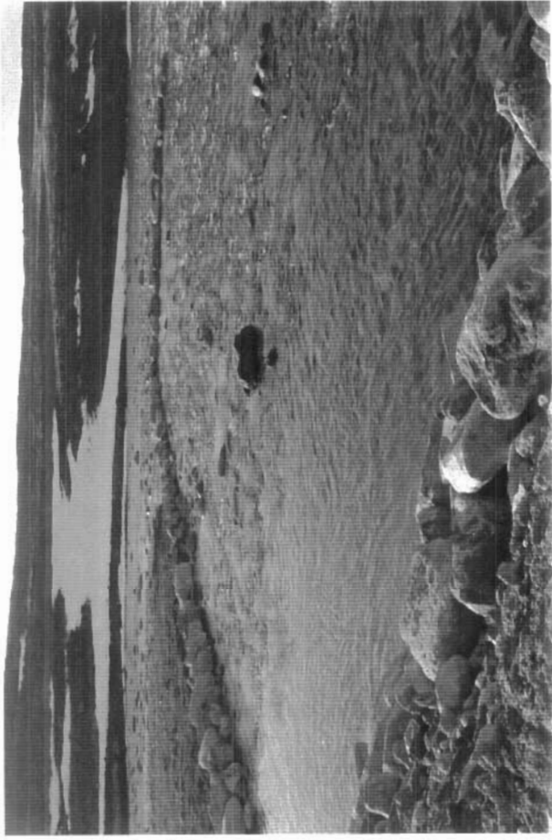
Plate 10 Second Bridge (Alliarusiq River), 30 June 2002. Spur dyke below bridge during high flow. Note: spur dyke is effective during this time period and has created a backwater holding area (bottom left).
