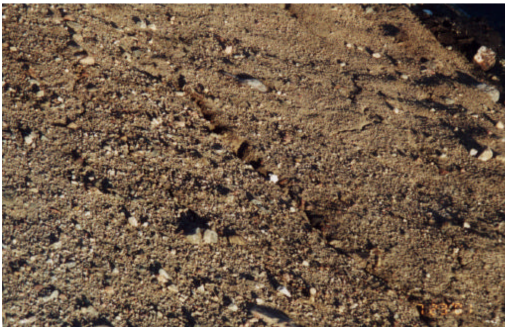
Photo 2 Longitudinal cracking along lagoon.
