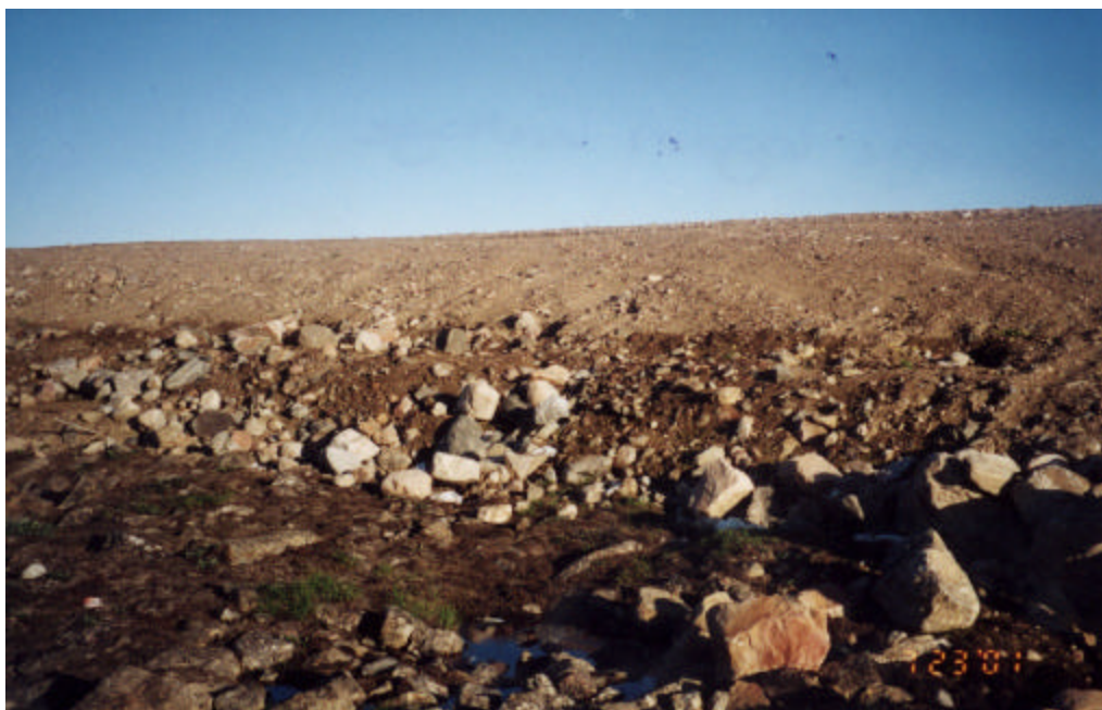
Photo 1 Liquid seeping from the north berm.
