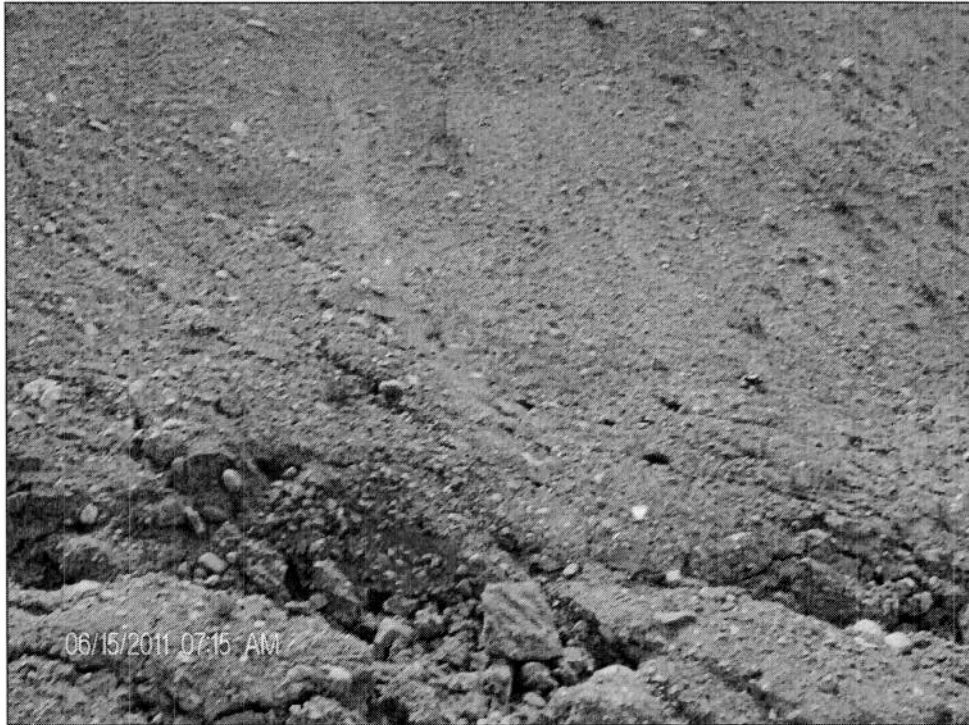
Photo 11: Longitudinal cracks in west half of the north berm close to toe of the berm.
