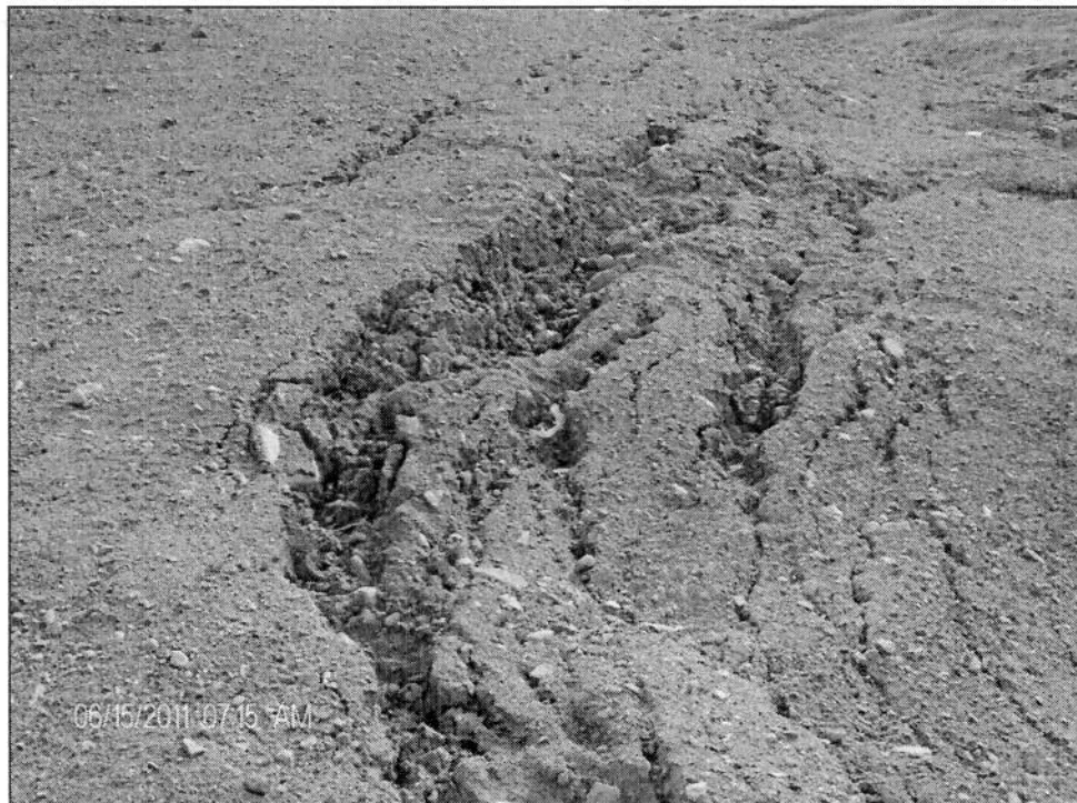
Photo 12: Longitudinal cracks in west half of the north berm close to toe of the berm.
