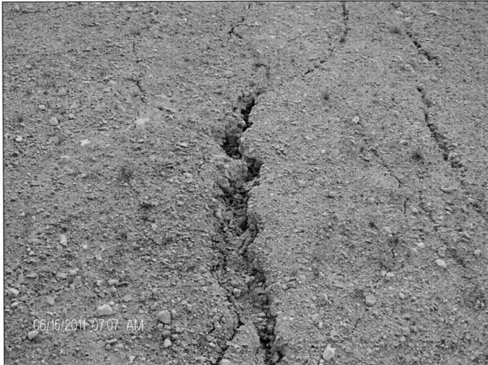
Photo 7: Longitudinal cracks in north berm extending from emergency flow to mid length of berm.
