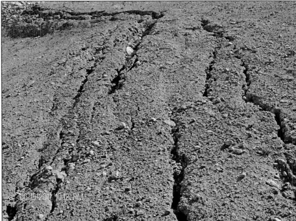
Photo 13: Longitudinal cracks in west half of the north berm close to toe of the berm.
