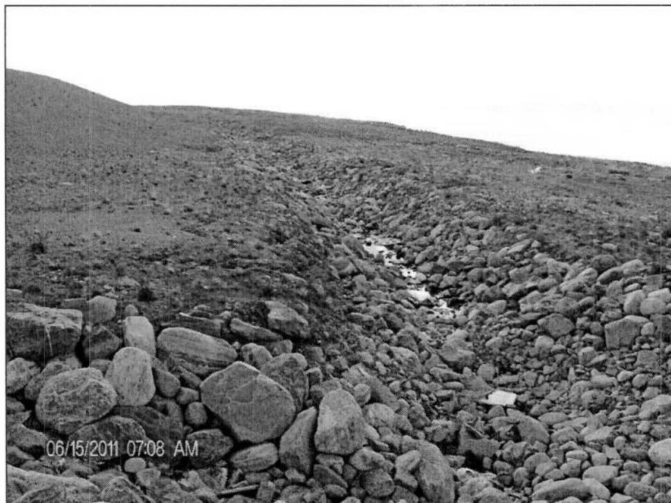
Photo 18: Drainage ditch at toe of north berm.
