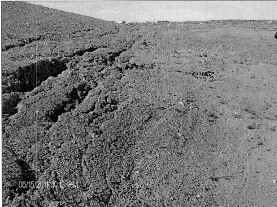
Photo 15: Longitudinal cracks in west half of the north berm close to toe of the berm.
