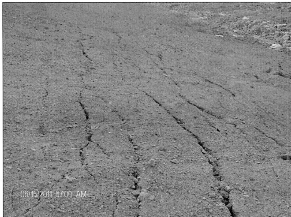
Photo 6: Longitudinal cracks in north berm extending from emergency flow to mid length of berm.
