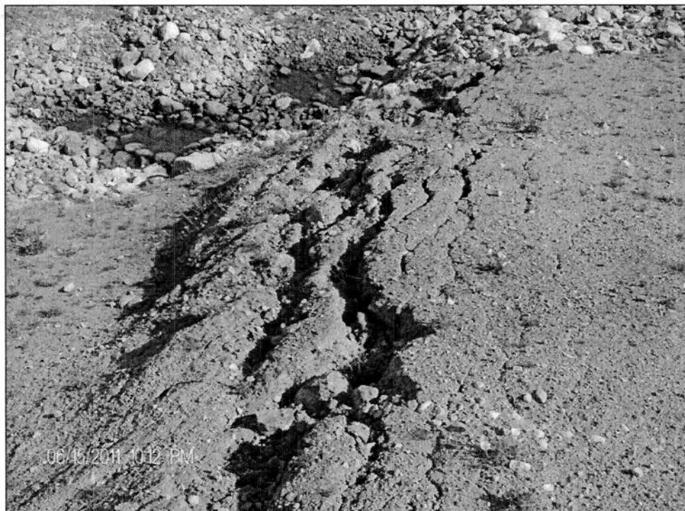
Photo 14: Longitudinal cracks in west half of the north berm close to toe of the berm.
