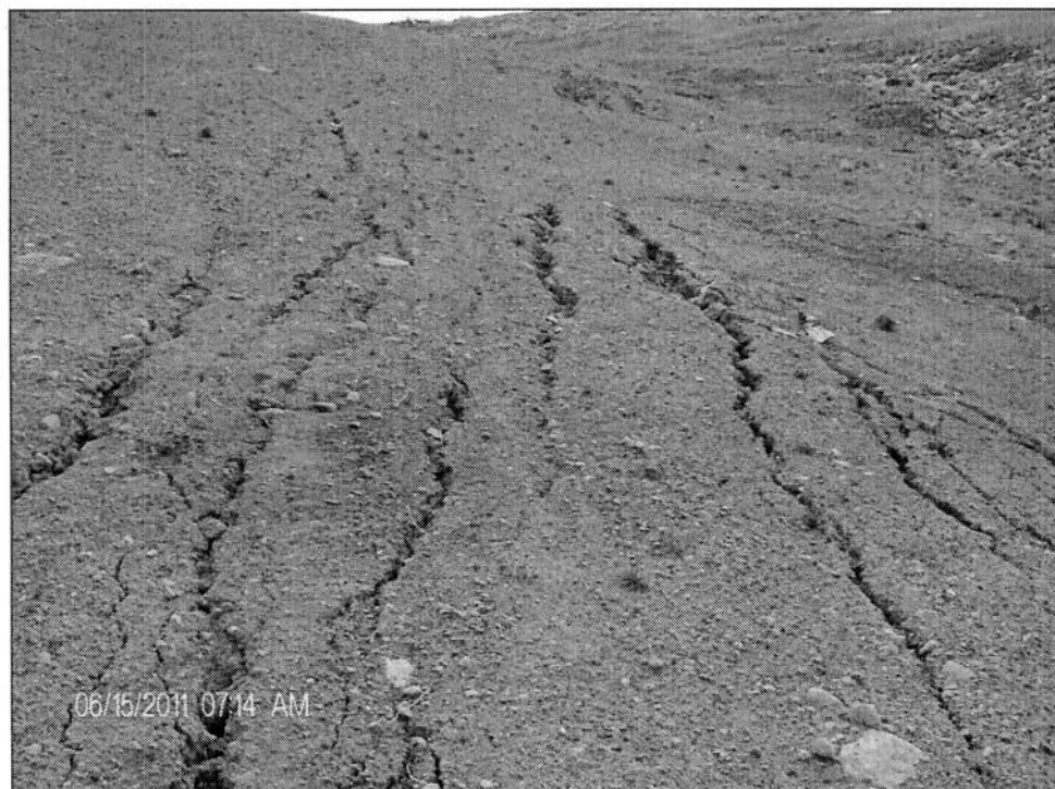
Photo 8: Longitudinal cracks in west half of the north berm close to toe of the berm.
