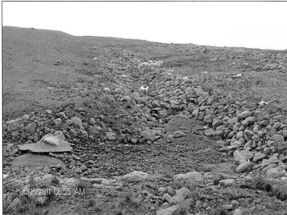
Photo 17: Drainage ditch at toe of north berm.
