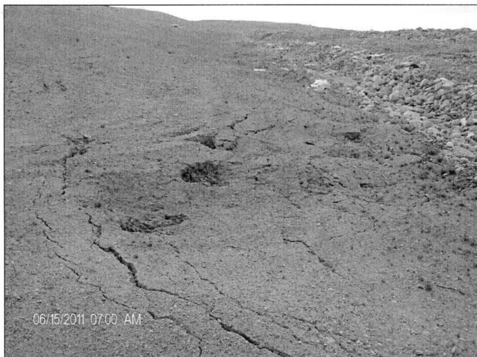
Photo 4: Longitudinal cracks in north berm extending from emergency flow to mid length of berm.
