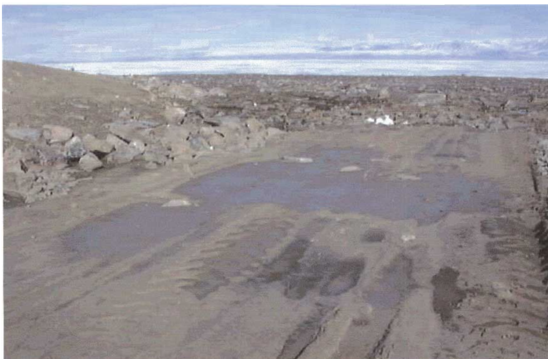
figure 3. Seepage from the NE corner of the sewage lagoon; 2001/06/26.
