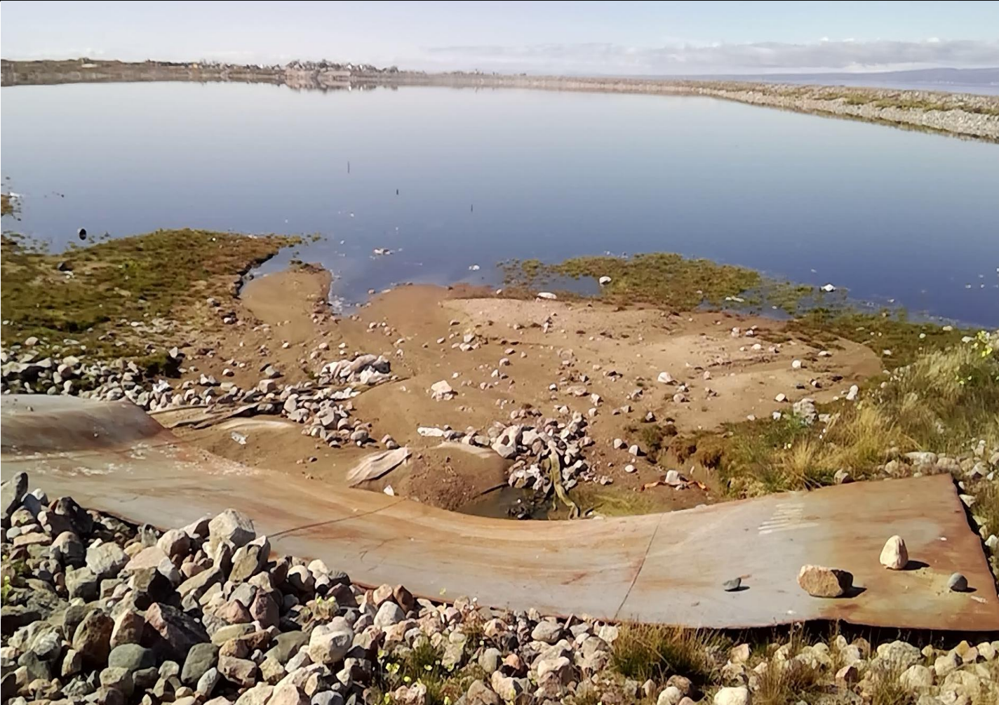
Description: The leak in the sewage lagoon appears to be under the metal slab.
