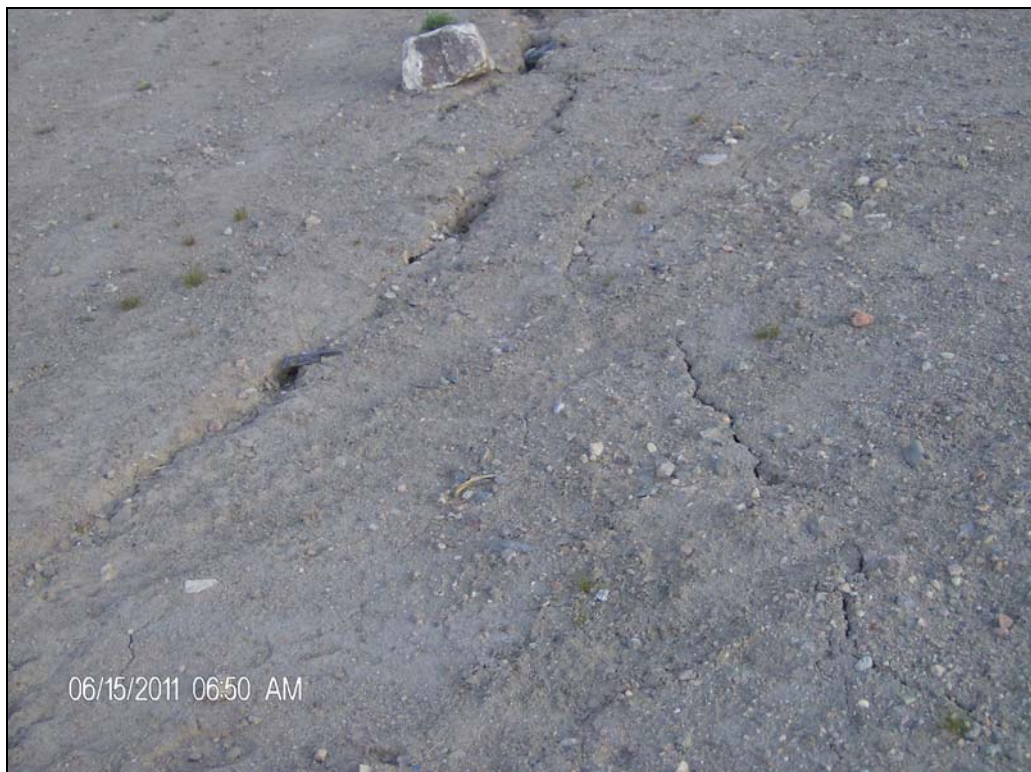
Photo2 : Longitudinal cracks in north berm at east end close to toe of berm.
