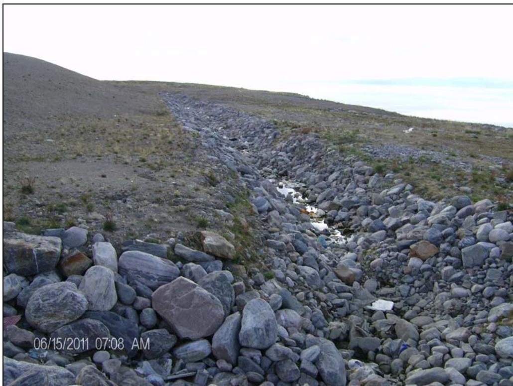
Photo 18: Drainage ditch at toe of north berm.
