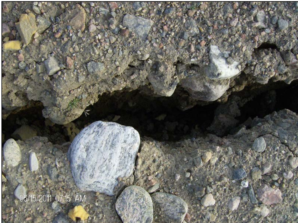
Photo 9: Longitudinal cracks in west half of the north berm close to toe of the berm.
