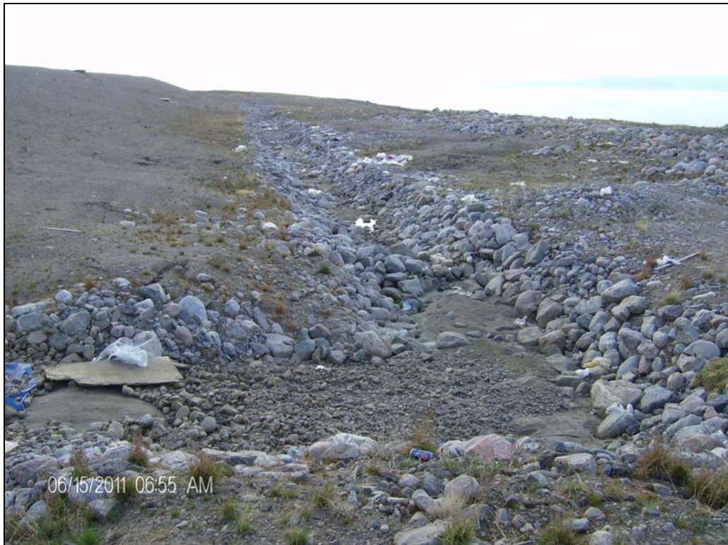
Photo 17: Drainage ditch at toe of north berm.
