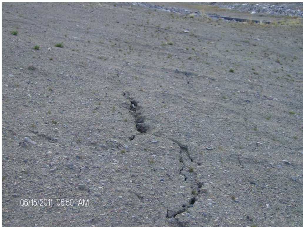
Photo 1: Longitudinal cracks in north berm at east end close to toe of berm.
