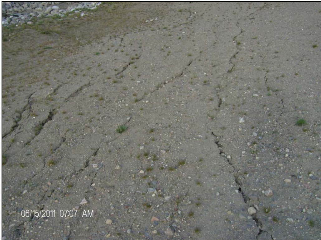
Photo 5: Longitudinal cracks in north berm extending from emergency flow to mid length of berm.
