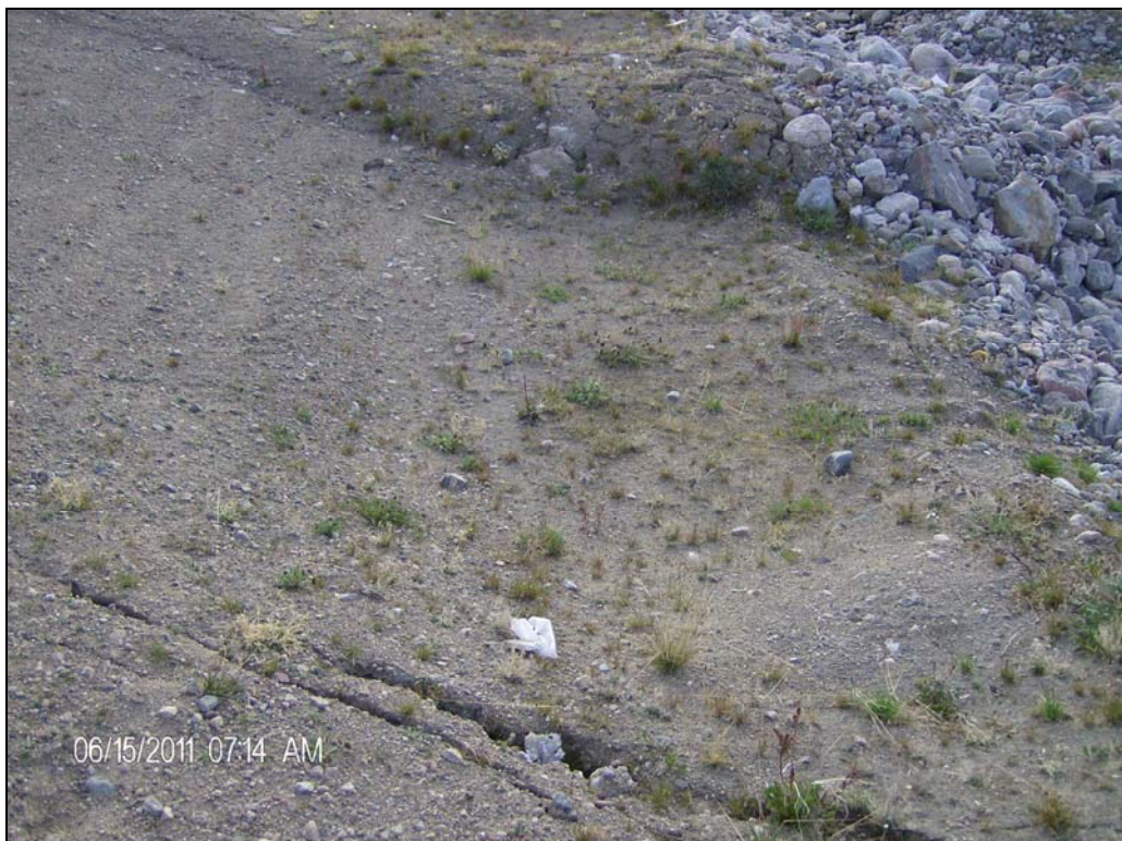
Photo 10: Longitudinal cracks in west half of the north berm close to toe of the berm.
