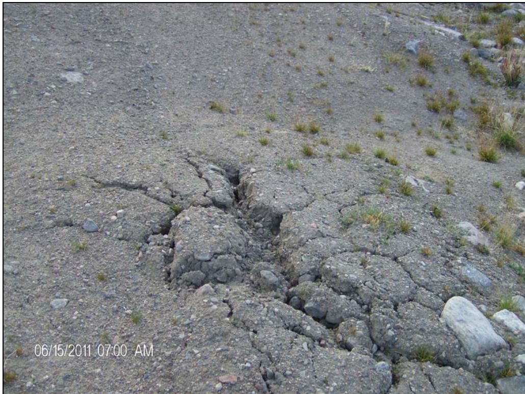
Photo 3: Longitudinal cracks in north berm extending from emergency flow to mid length of berm.
