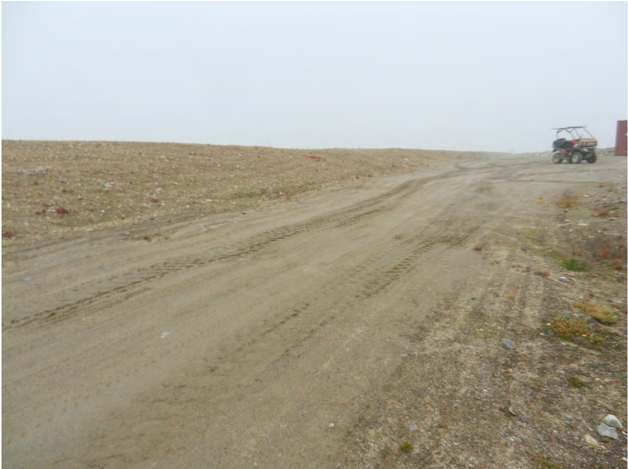
Photograph 2 – Settlement across access roadway adjacent to easternmost berm of lagoon 5
