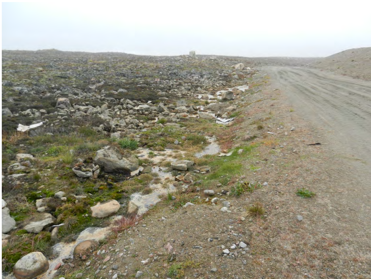
Photograph 1 – Leakage area identified by GN-CGS at easternmost berm; facing south (liquid level on 23 August)
