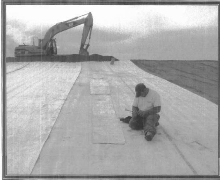
Photo # 1. Laying down Bentomat ST GCL
