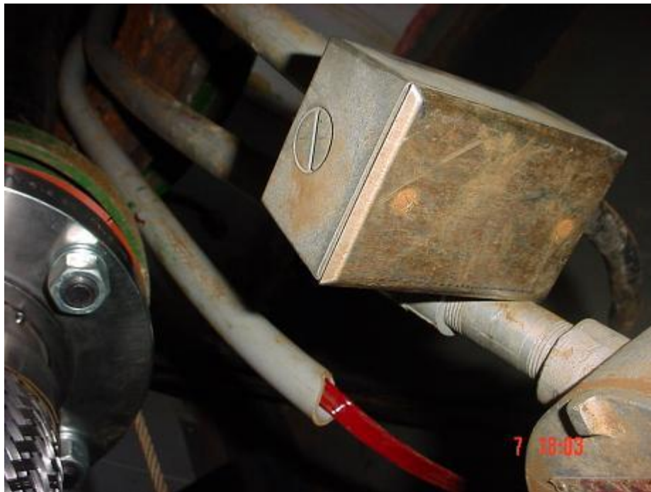
Figure E-10: Rusting Screws at Pump Chute Box
