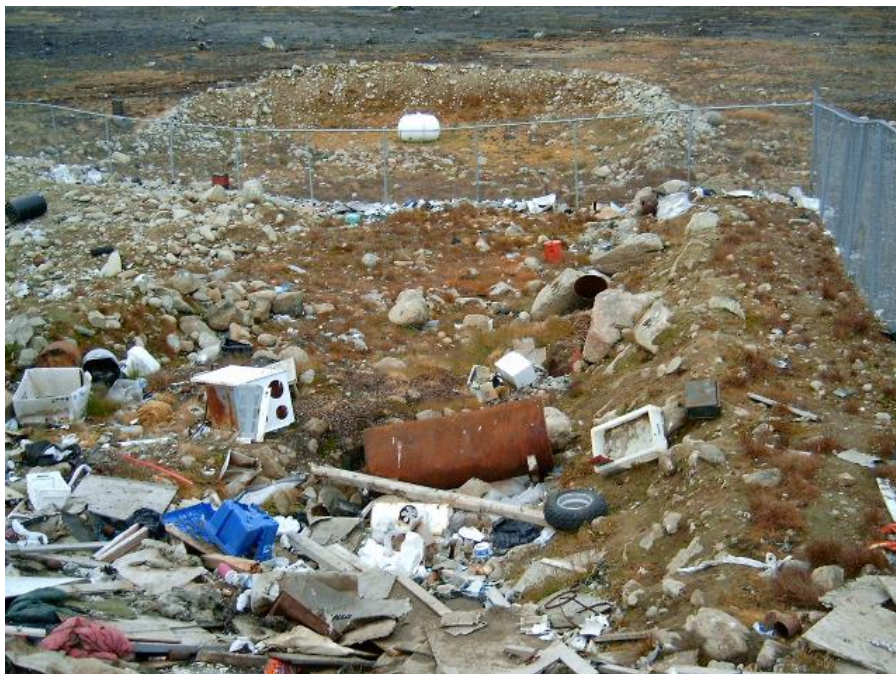
Photo 10 Dry leachate collection pond at base of landfill.
