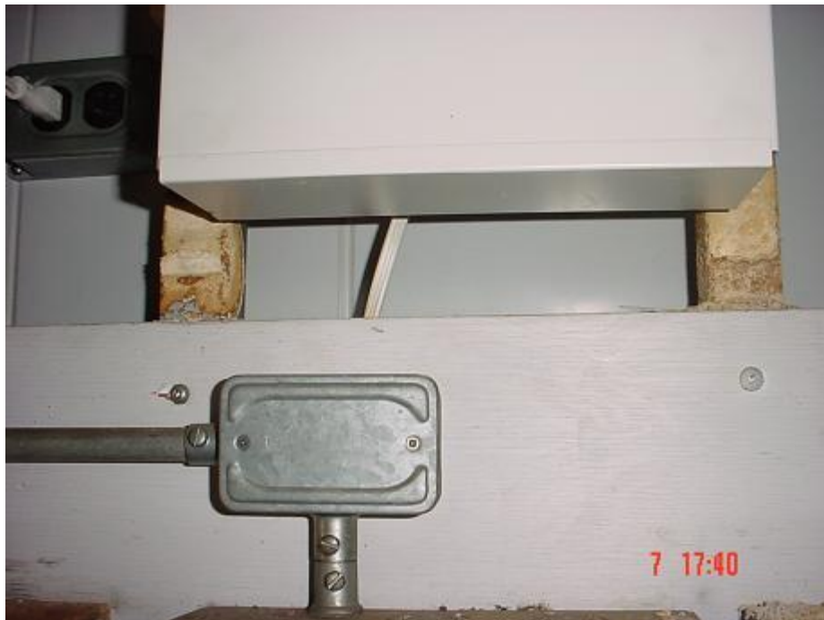
Figure E-16: Corrosion Under Battery Pack
