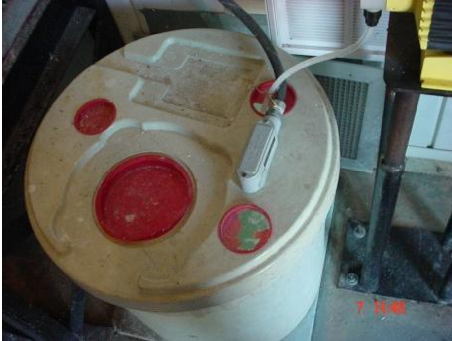
Figure E-13: Broken Lids on Chlorine Mixing Tanks
