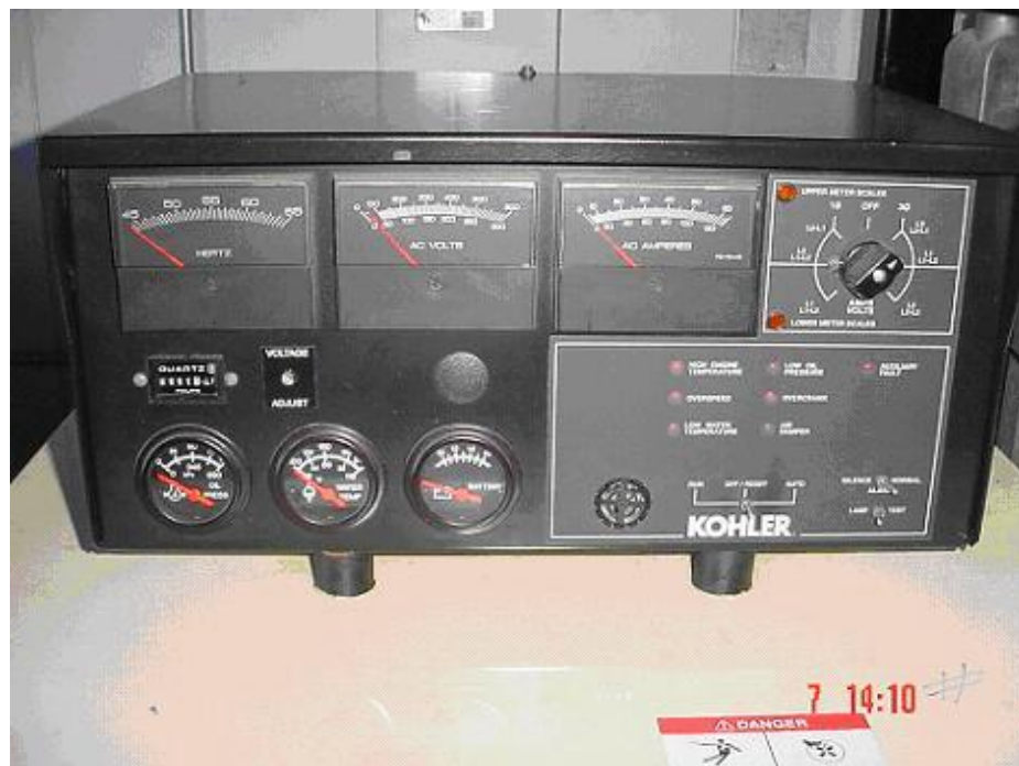
Figure E-2: Generator Control/Indication Panel
