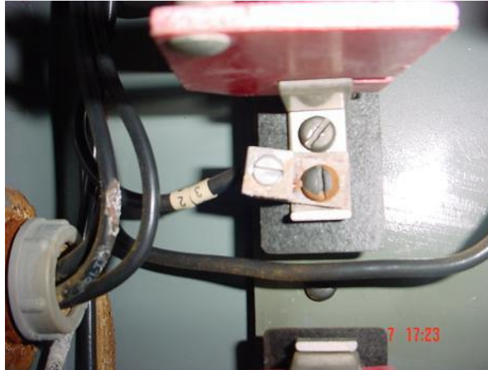
Figure E-17: Dust Build-Up on Lugs
