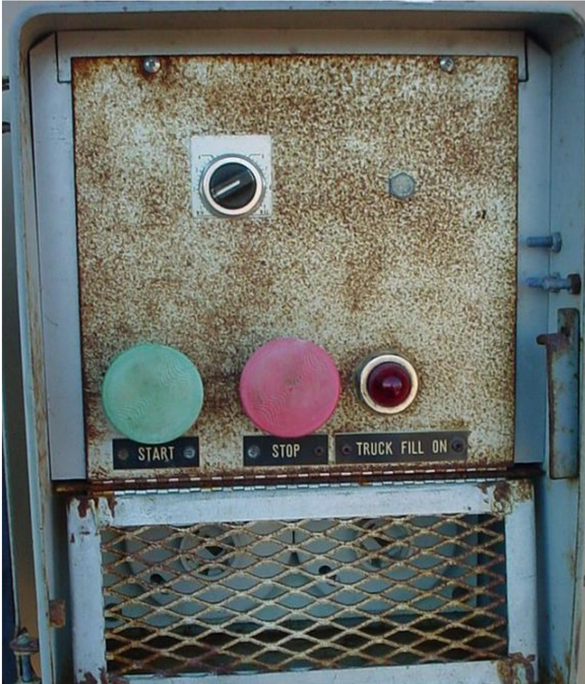
Figure E-8: Truck Fill Controls
