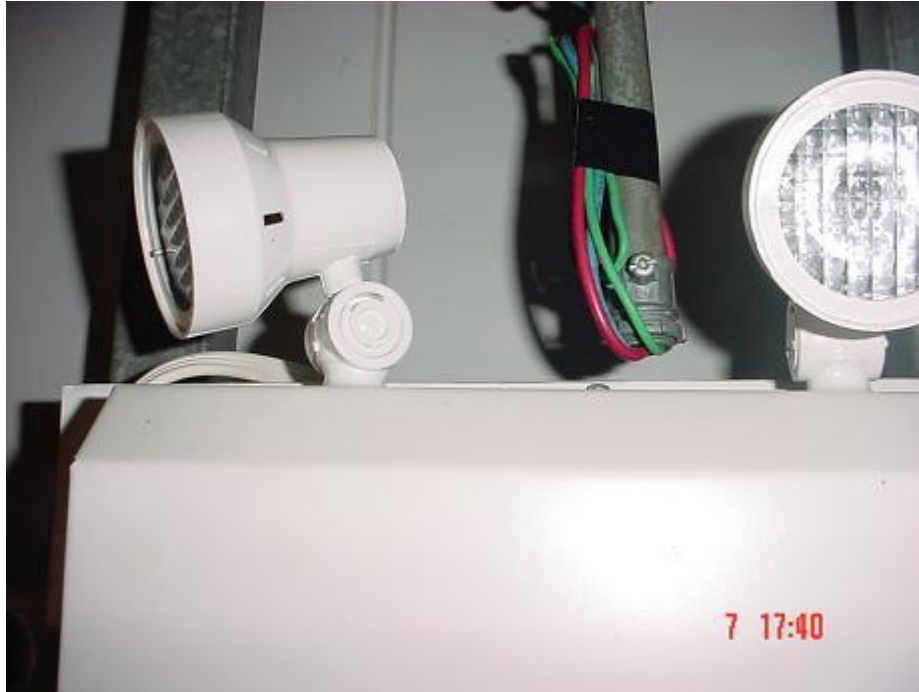
Figure E-15: Unused feeders from Indication Panel
