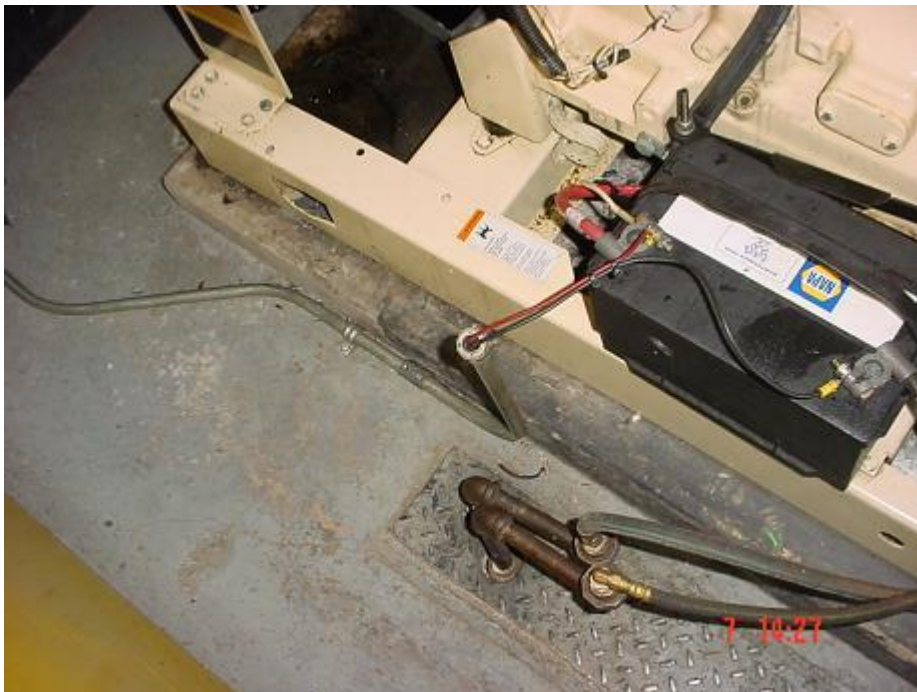
Figure E-14: Generator Battery Connection
