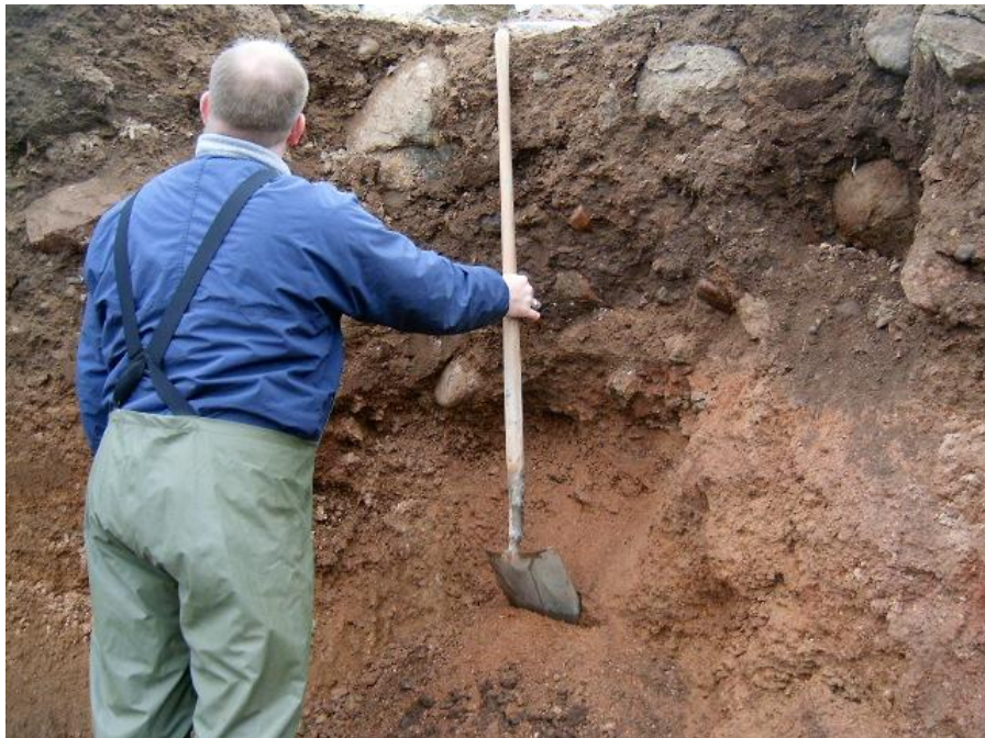
Photo 4 Typical excavation face at the quarry site. Permafrost at approximately 2.0 m below surface.
