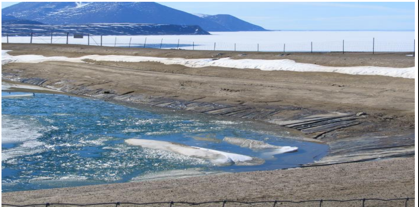
Water Storage Reservoir
