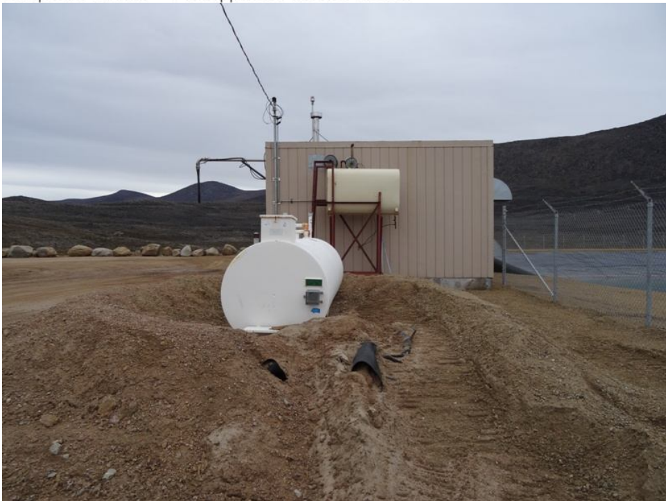
Figure 11 Pumping/ Transfer Station with two fuel tanks and crushed berm wall
