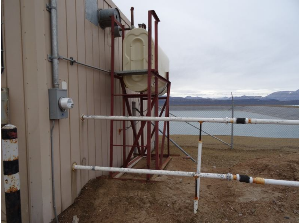
Figure 10 Pump Station - Single walled piping from 1000 gal tank
