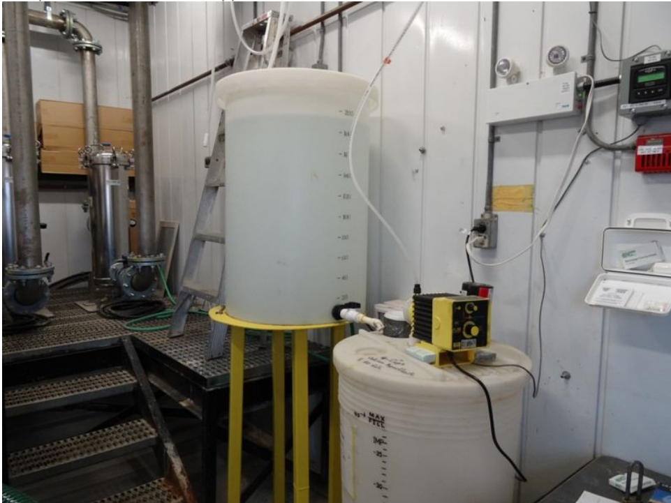
Figure 14 Chlorination system
