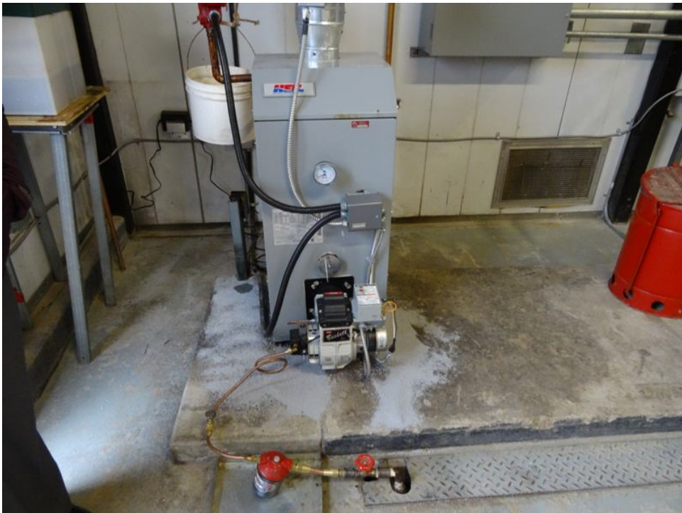
Figure 13 Fuel leaks inside pumping station
