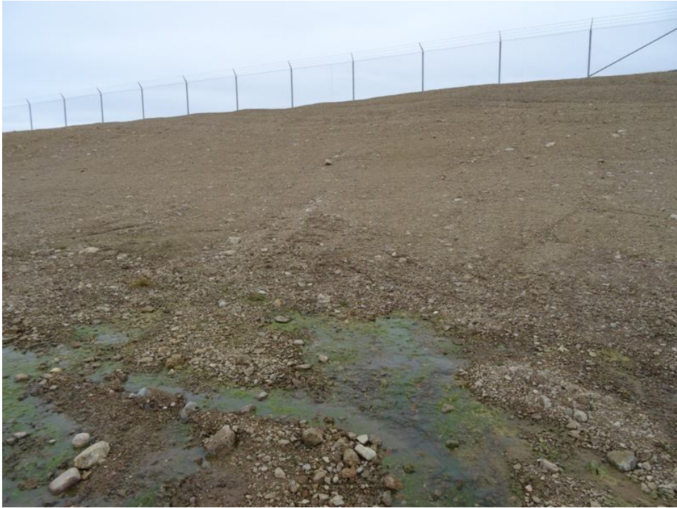
Figure 7 Reservoir - flow from toe
