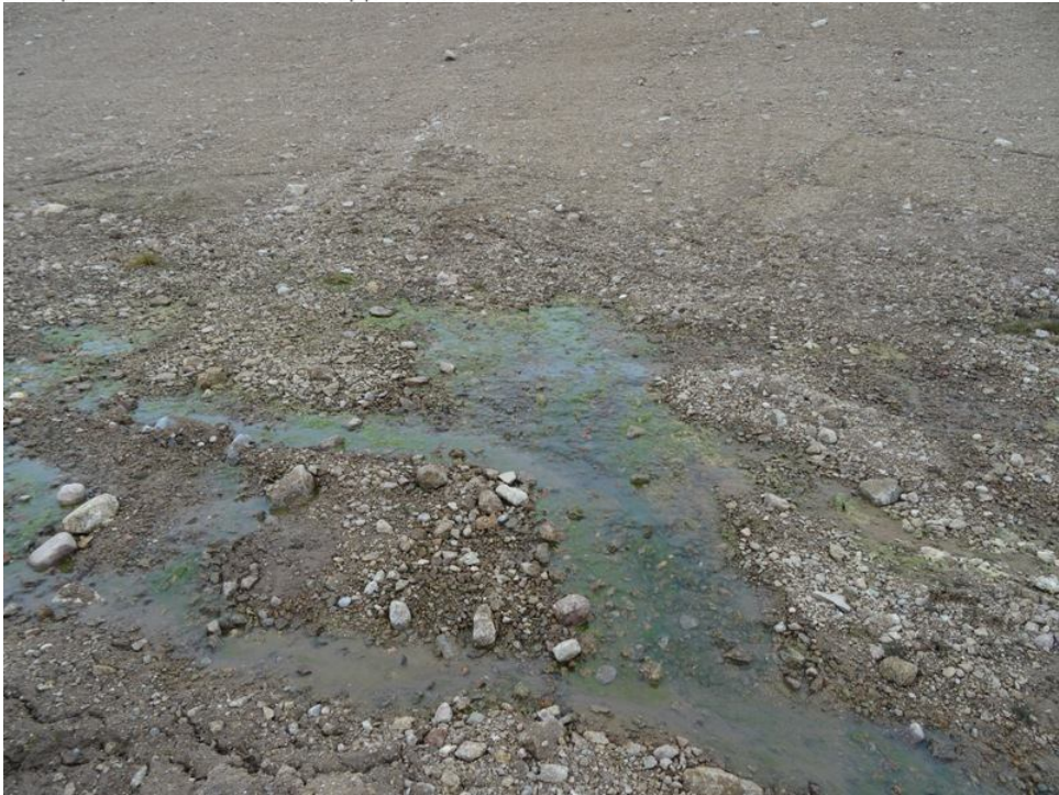
Figure 8 Reservoir – water from under toe
