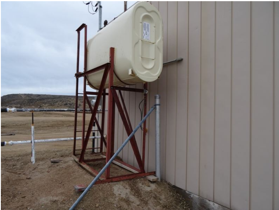
Figure 12 Pump Station with household fuel tank - unsecured to building
