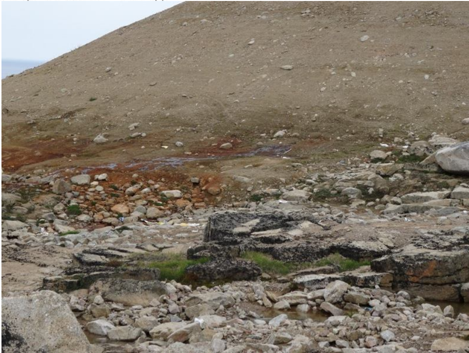
Figure 35 Flow from toe of new lagoon cell
