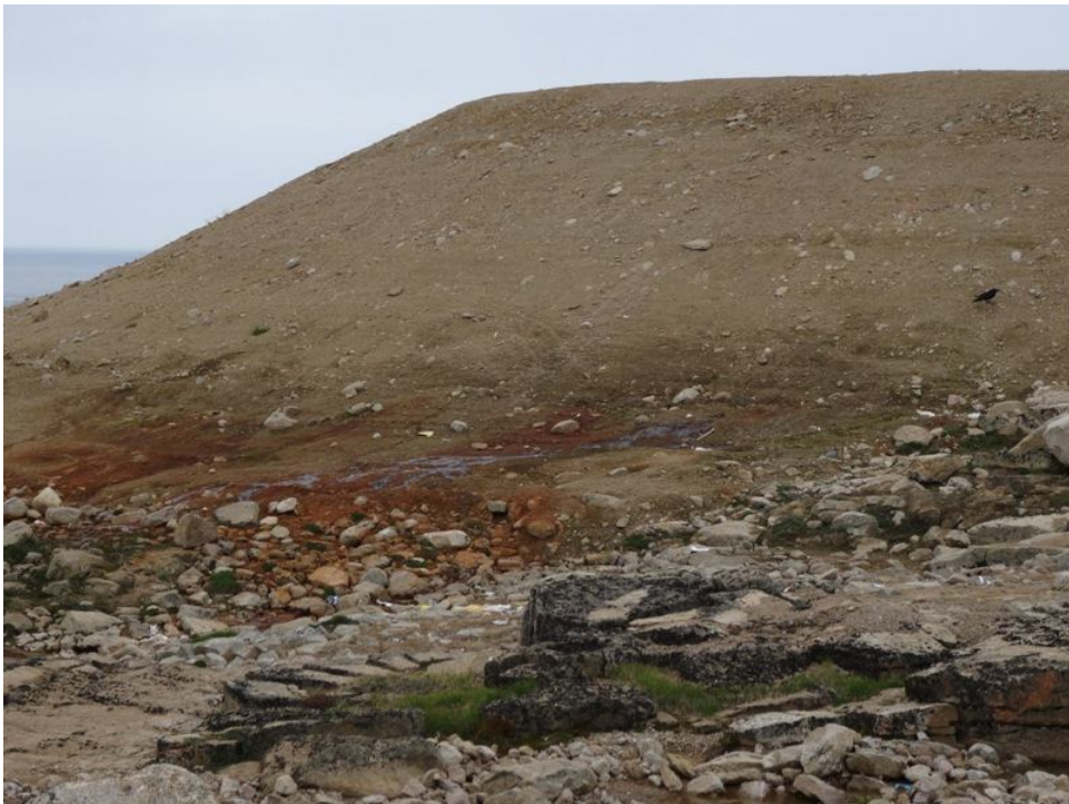
Figure 34 Flow from Toe of new lagoon cell
