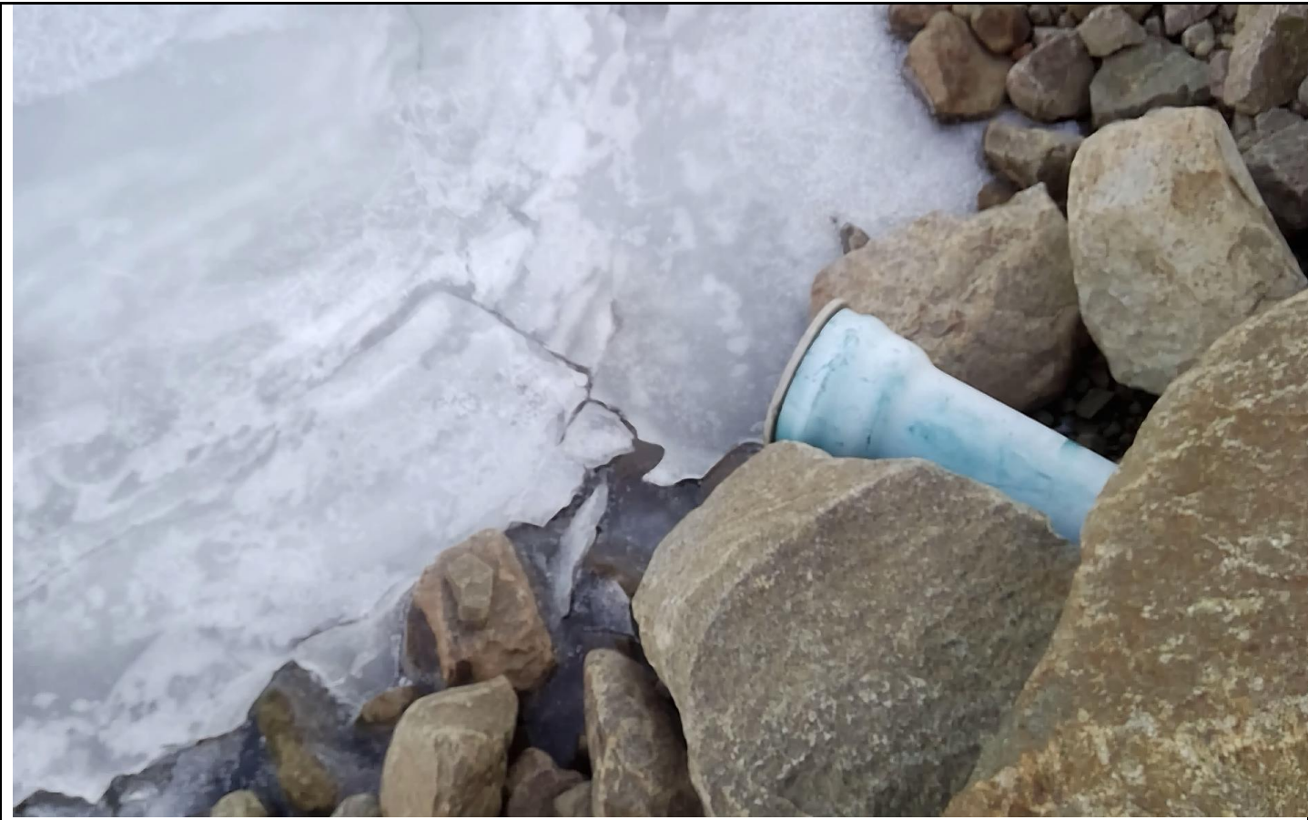
Description: water intake pipe. More than 50% below the water table.
