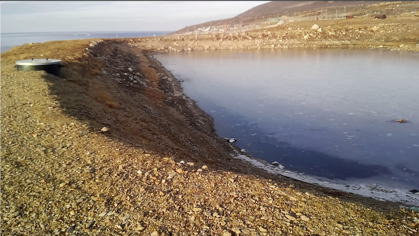
Description: Signs of windblown garbage in Waste Water Treatment Facility – Decanting Pipe appears above the lagoon waste water table. Freeboard appears to be above the 1 metre freeboard. Some free blown garbage observed in the lagoon.
