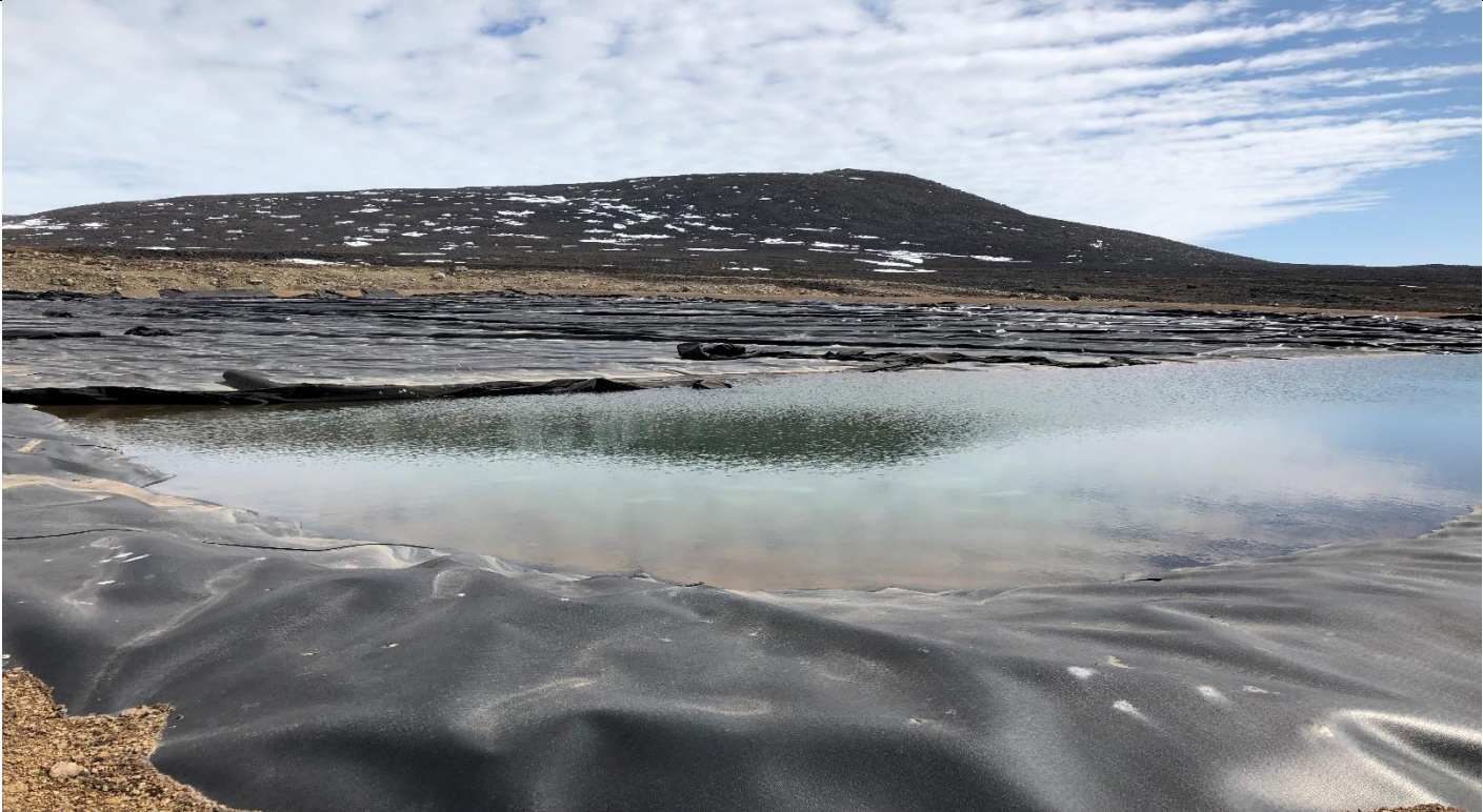
Description: Water in the soil remediation berm. No signs of activity in 2021, but the accumulation of water in the berm indicates the berm isn't damaged.
