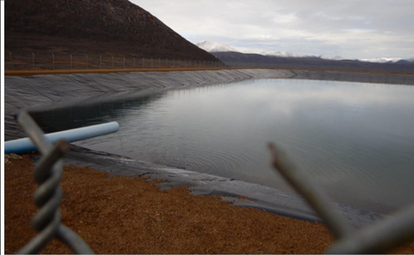
Description: Water Reservoir – intake pipe from water withdrawal location at Tulugak River. Uncontrolled withdrawal of water from the water source
