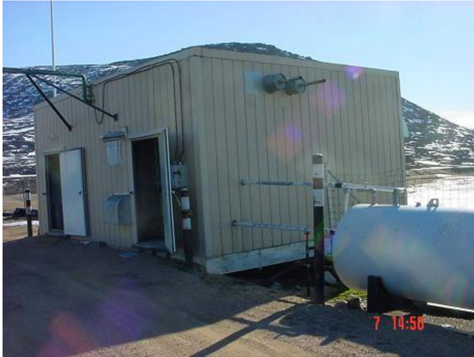
Figure E-1: Truck Fill Station (Pump Room on Left, Generator Room on Right)
