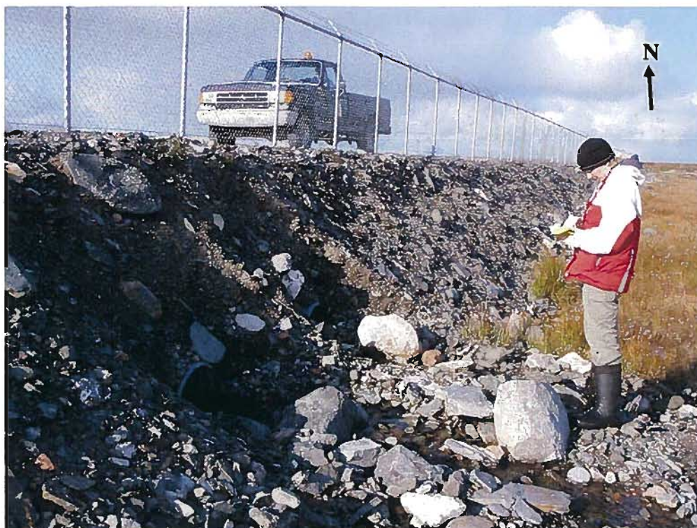
Photo 7: Culvert on east side of landfill, discharge point.
