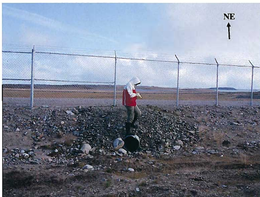
Photo 4: Culvert on west side of landfill
