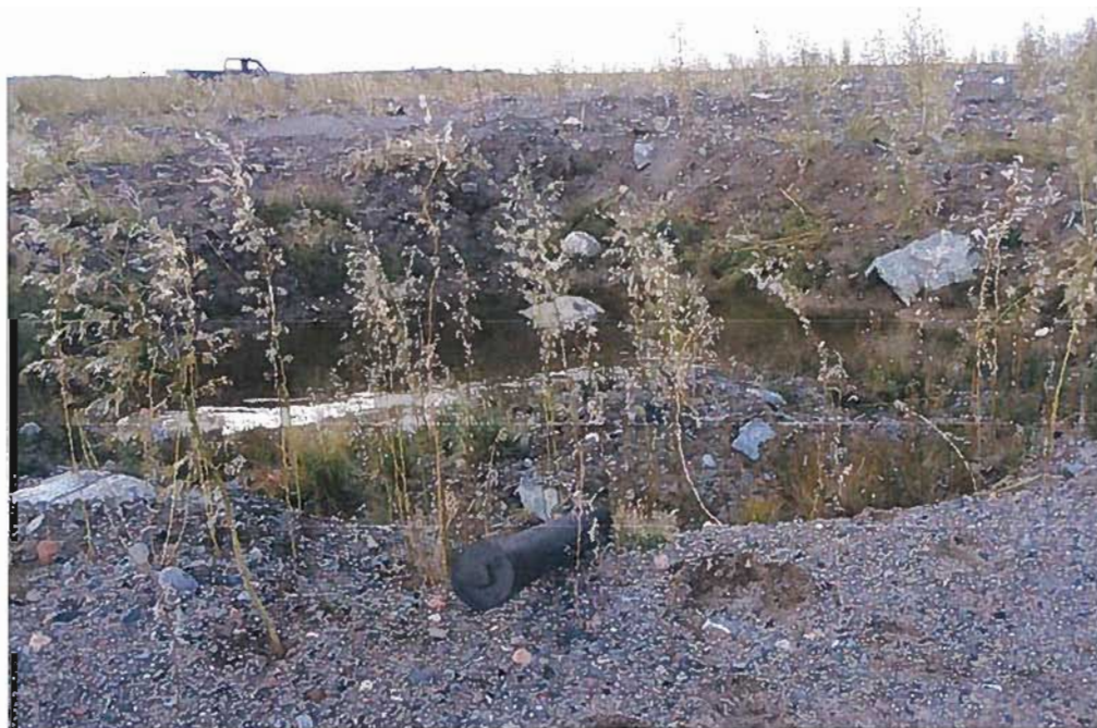
Photo 16: Leachate drainage pipe, looking northwest.
