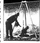
body harness. Where primary access is unavailable, a grum winch can be used as primary access into the confined space. In addition to the drum winch, a retrieval lifeline is used as a secondary backup for fall protection and rescue. The drum winch can be used to lower and raise materials after the worker has accessed the confined space, while still ensuring rescue in the event of an emergency.
