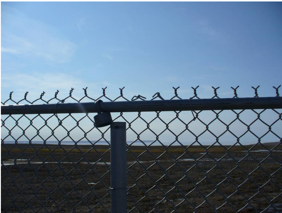
Figure 39: Disconnect top rail to line post at top of post.
