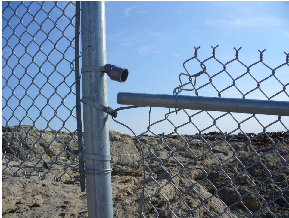
Figure 36: Top rail connection, disconnected.
