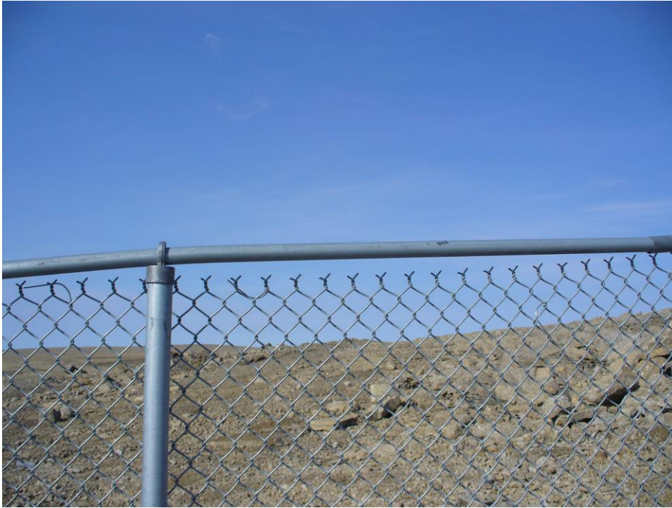
Figure 40: Chain link short from top rail.
