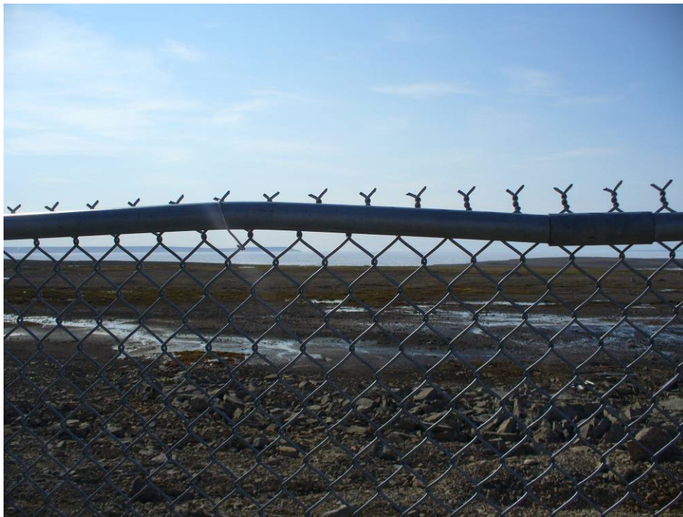
Figure 37: Localized bent top rail.
