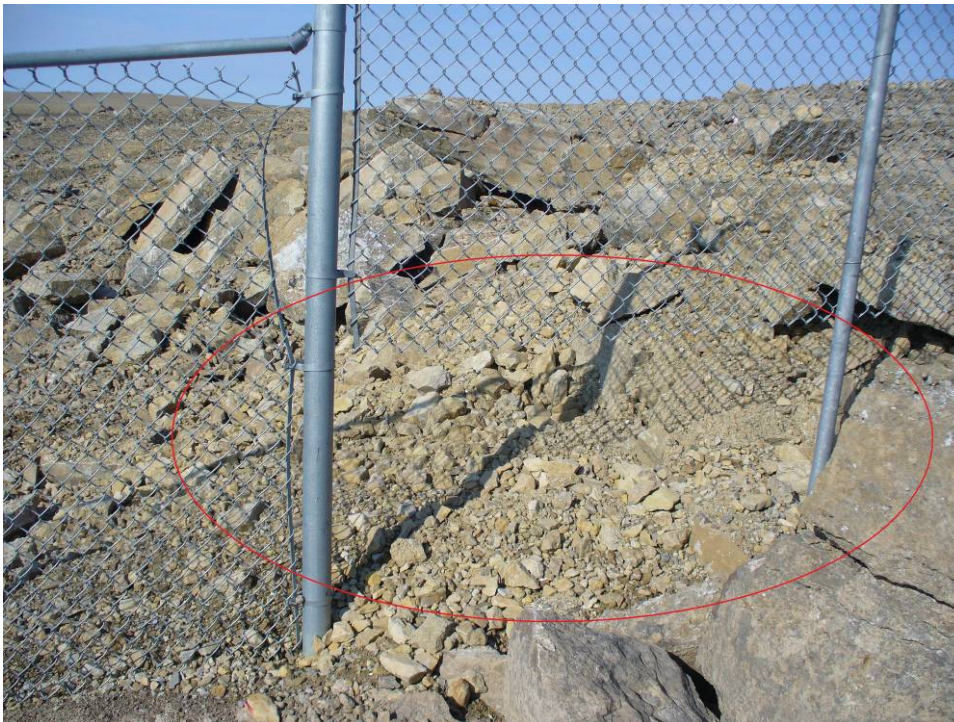
Figure 34: Gapping at base of fence based on terrain.
