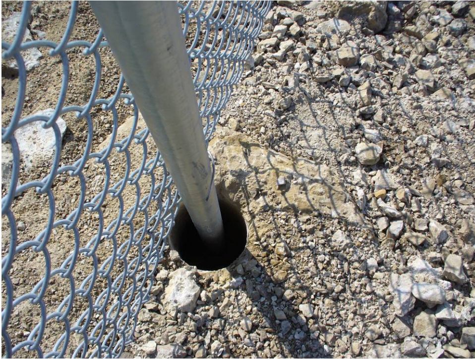
Figure 42: Drilled and embedded post lacking backfill to top of hole.
