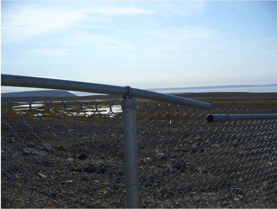
Figure 38: Localized disconnection of top rail at top rail sleeve.
