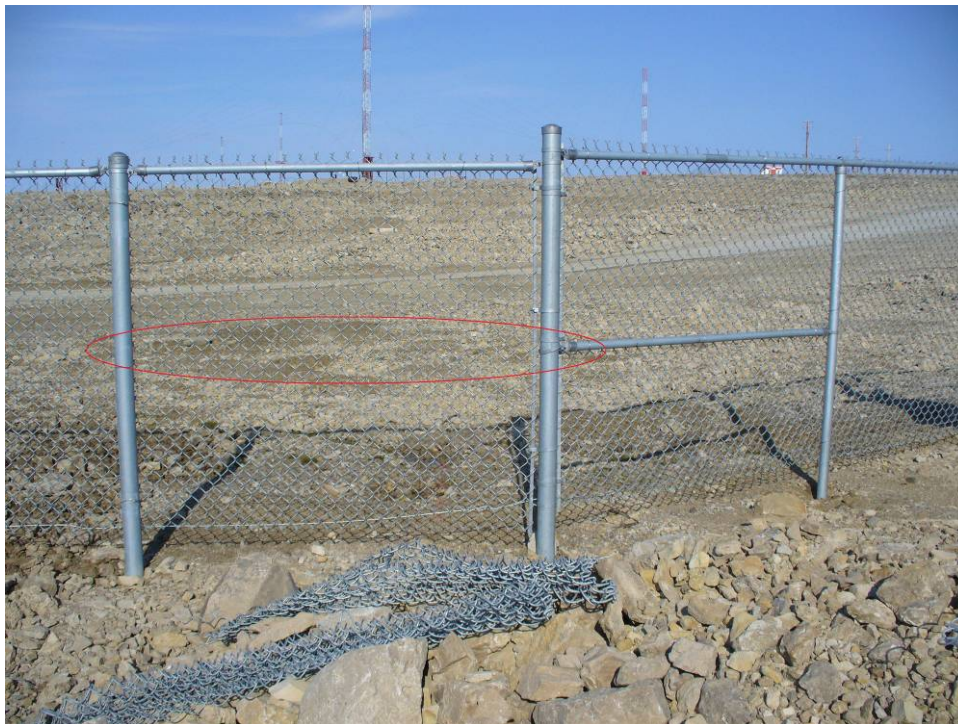
Figure 41: Potential location for addition of new bracing member.
