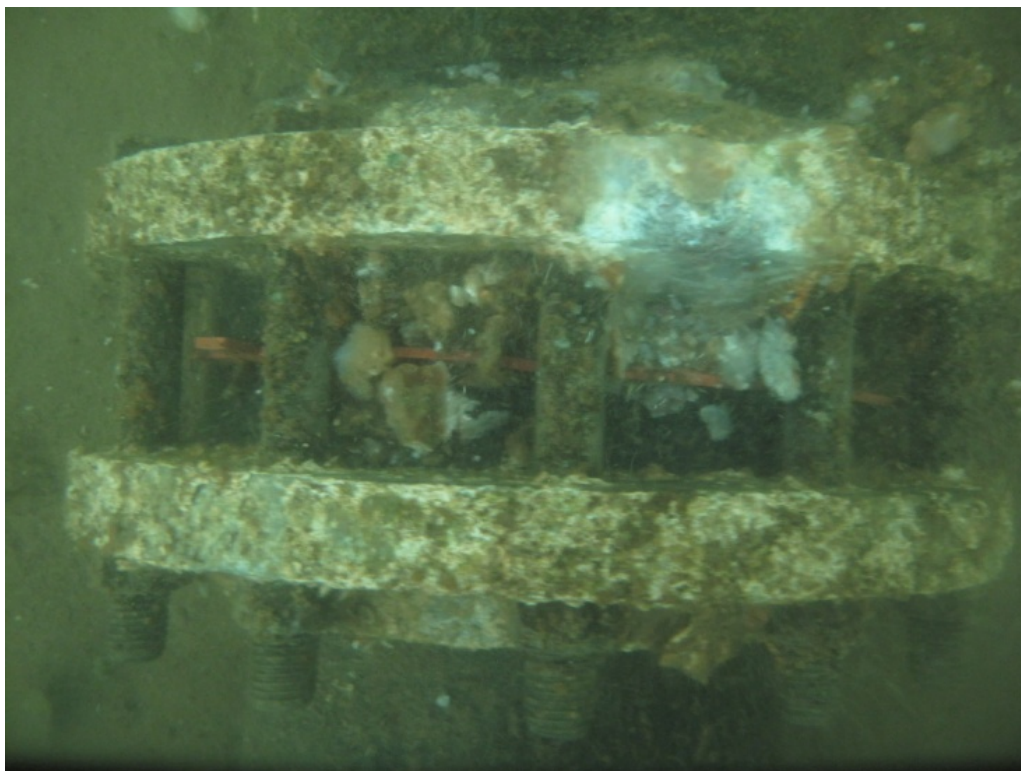
Photo 3: Typical Flanged Joint at Lateral
