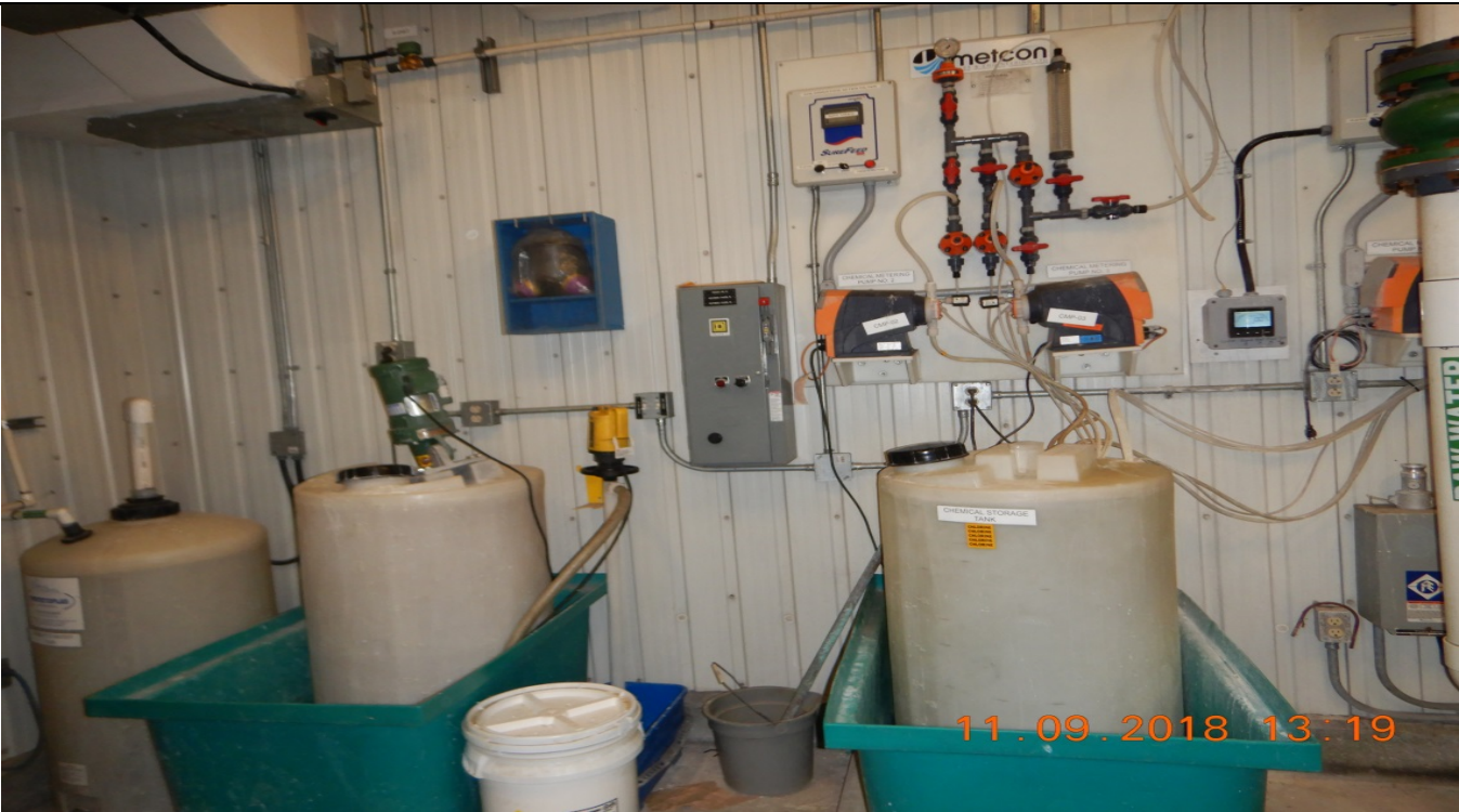
Description: Two Chlorine Mixing drums
