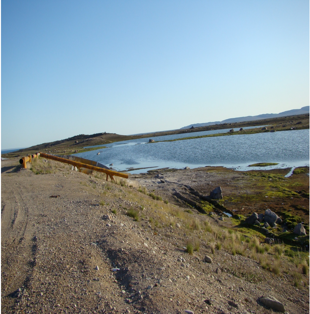
Picture 2: Taloyoak Sewage Lagoon. Secondary cell connected to a natural wetland for summer remediation of effluent.
