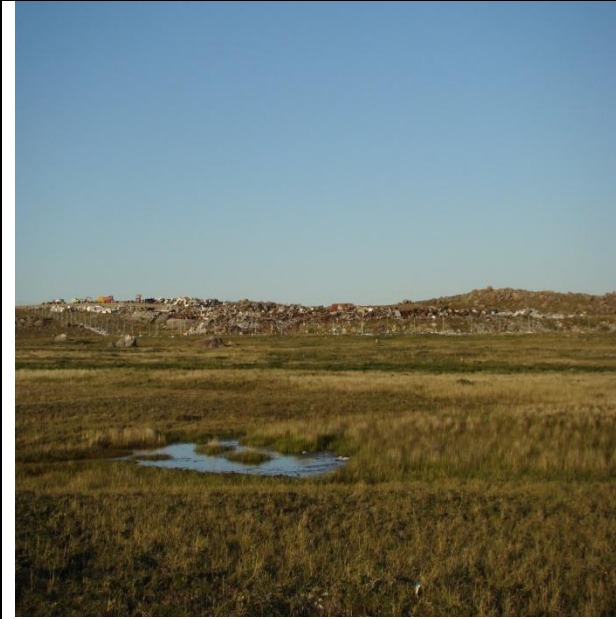
Picture 5: solid waste run-off storage sump
