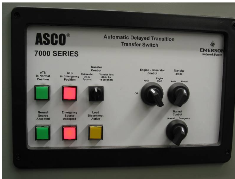
Figure 5: ATS control switches
