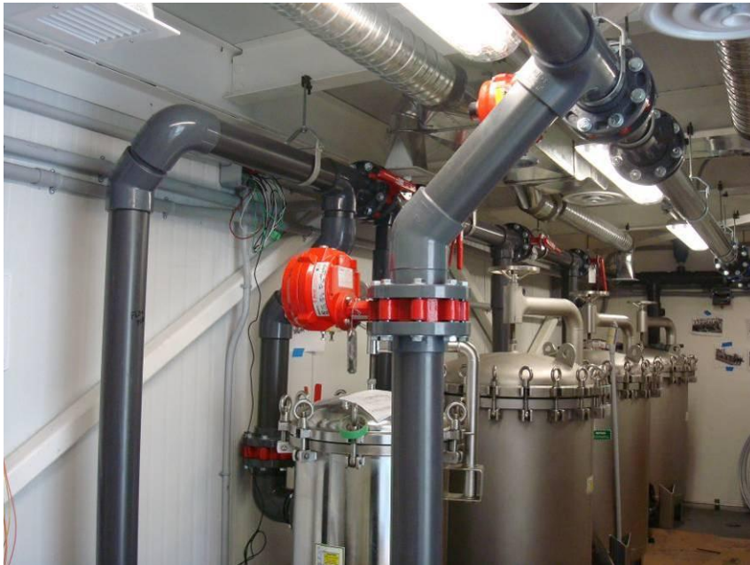
Fig. 1 Swing bolt cartridge filter housings.
