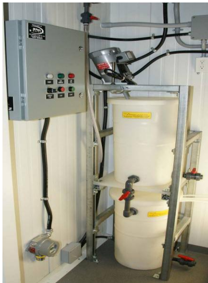
Fig.2 Calcium hypochlorite mixing arrangement.
