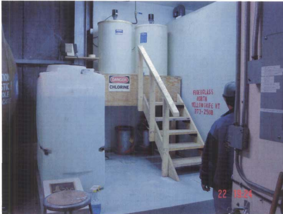
Photo # 3 Chlorination system in Water Treatment Plant.
