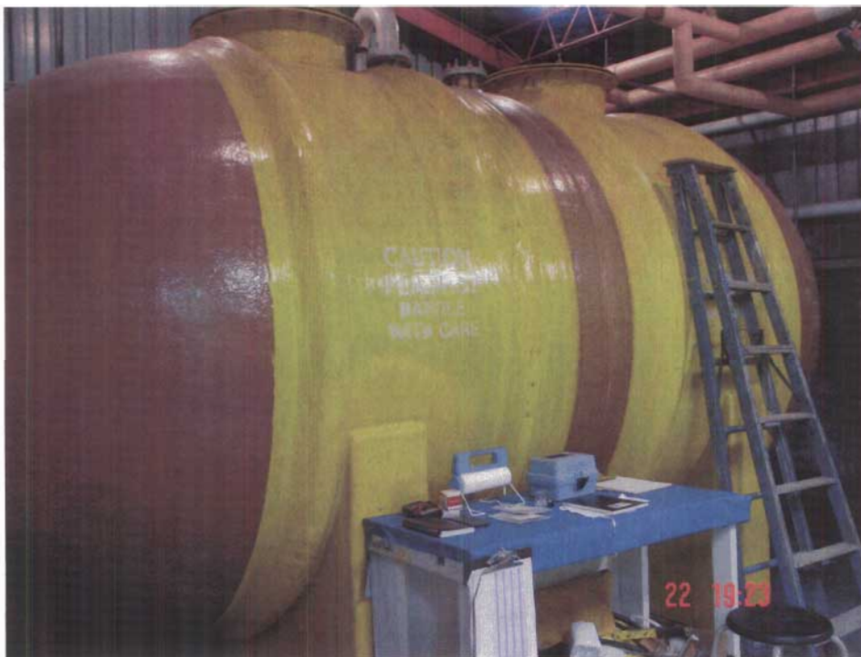
Photo # 4 One of 2 storage tanks for potable water in Water Treatment Plant.
