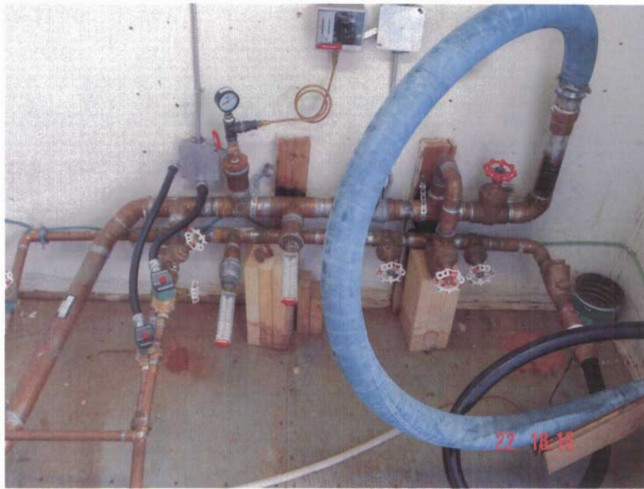
Photo # 1 Water Intake Facility interior piping for water truck filling.
