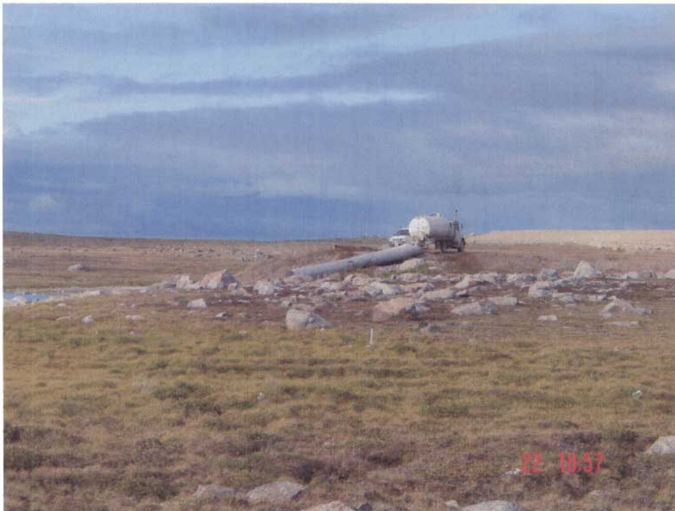
Photo # 10 Sewage Lagoon, sewage truck discharge structure.
