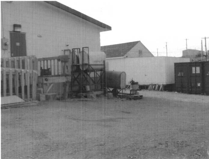
Photo 4. Fuel oil storage located well within 30 metres of the high water mark of the community potable water supply, note no berms.
