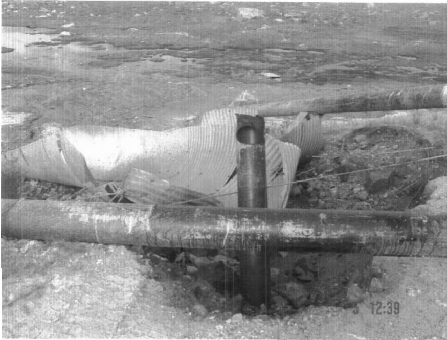
Photo 11. Erosion at sewage truck discharge structure.
