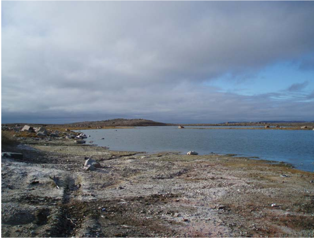
Photo 3. No berms surrounding the lagoon creating very little retention time.
