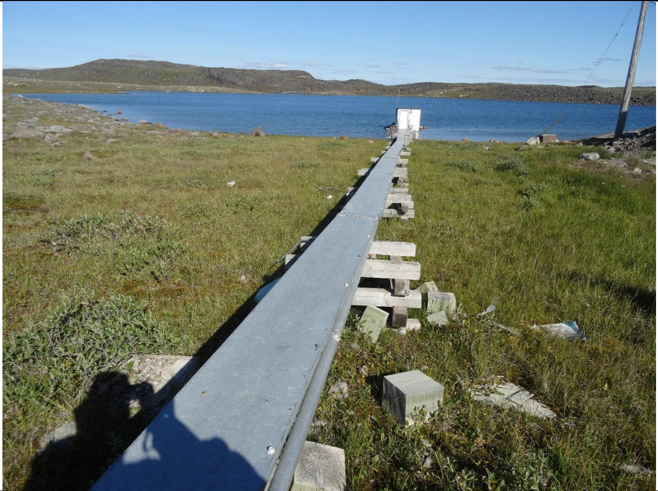
Description: Old Pump House and Utilidor System requiring Reclamation – View 1
