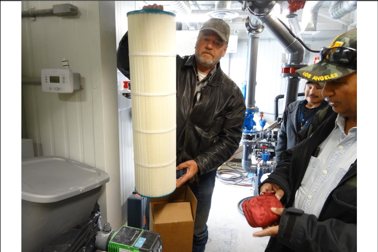
Description: Water Filters used in Canso Lake Intake Pump & Truck Fill Station that could be sent south for recycling
