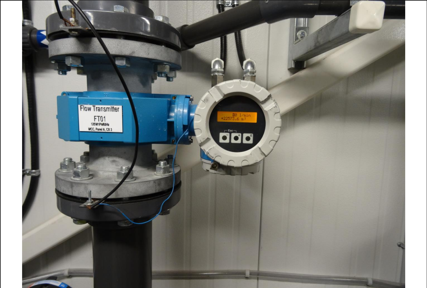
Description: Raw Water Intake Inline Flow Meter inside Canso Lake Intake Pump & Truck Fill Station
