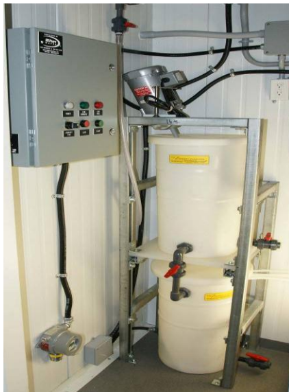
Fig.2 Calcium hypochlorite mixing arrangement.
