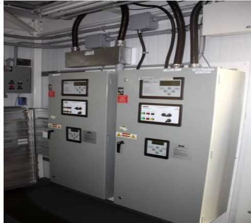
Figure 4: Automatic Transfer Switches ATS1 (“Load Switch”) on the right, ATS2 (“Power Switch”) on the left
