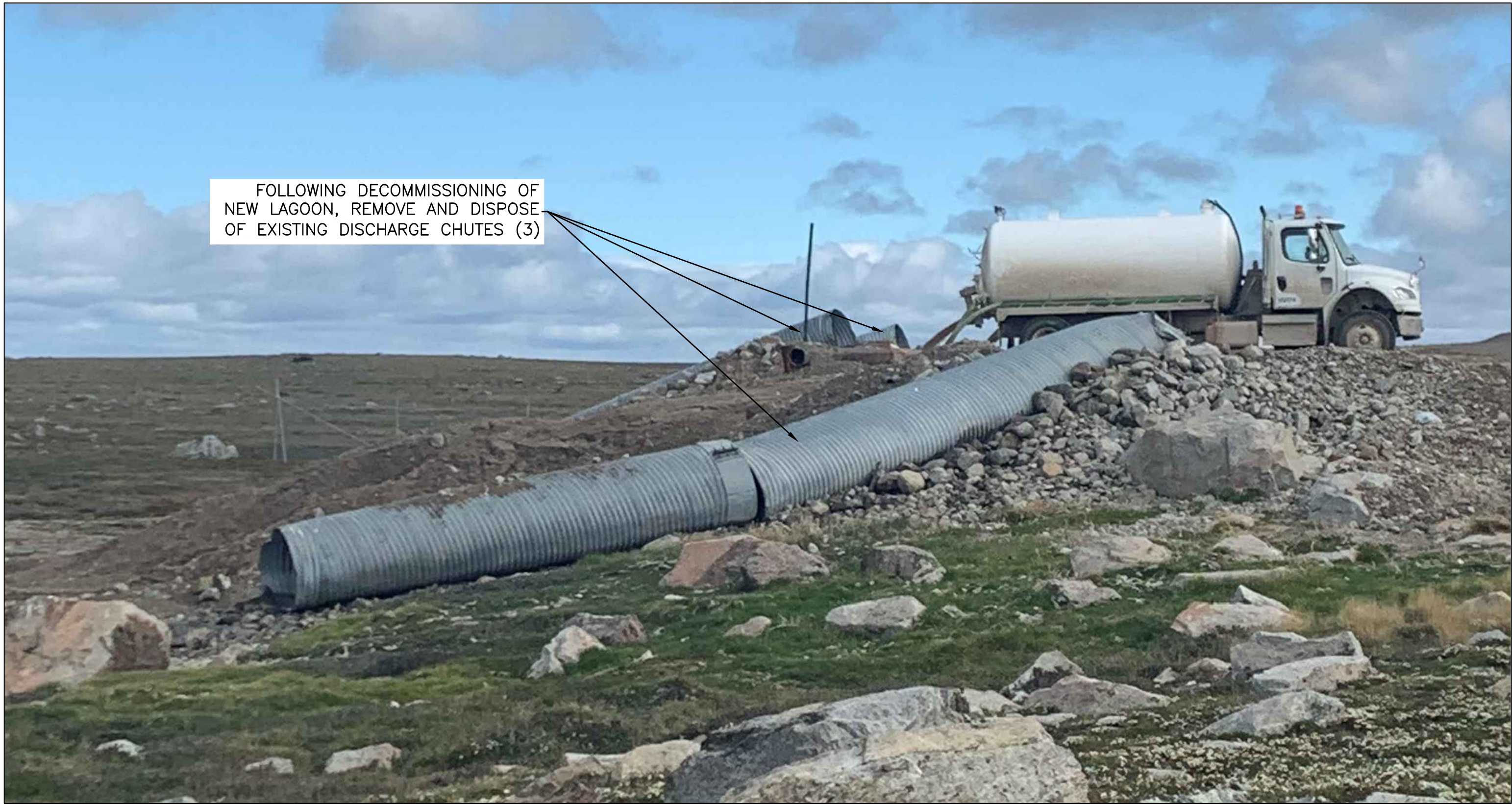
DETAIL "J1" REMOVAL OF EXISTING DISCHARGE CHUTES N.T.S.
