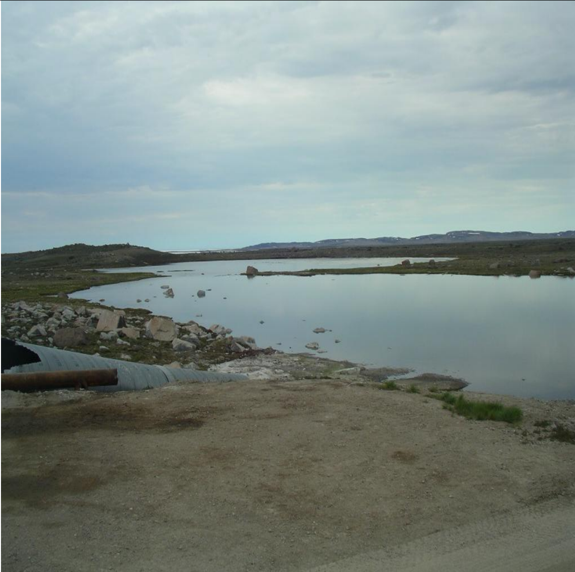
Taloyoak sewage facility: Two cell natural Lake sewage lagoon with natural berm in between
