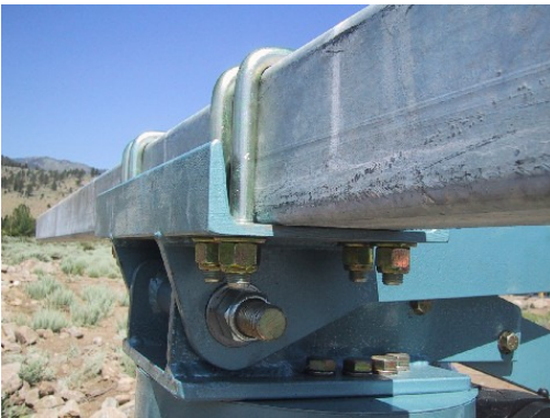
TIGHTEN NYLOCK 5/16" U-BOLT NUTS EVENLY .
