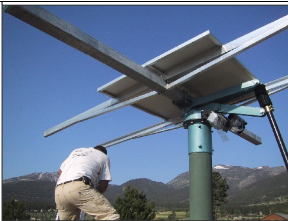
Module Rail & Support Angle Detail From the bottom
