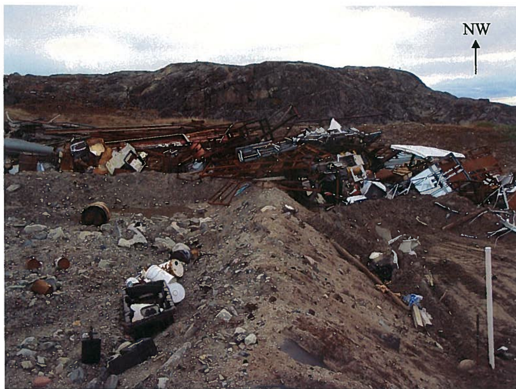
Photo 19: Berm around landfarm with liner showing through and metal waste overflowing onto landfarm.
