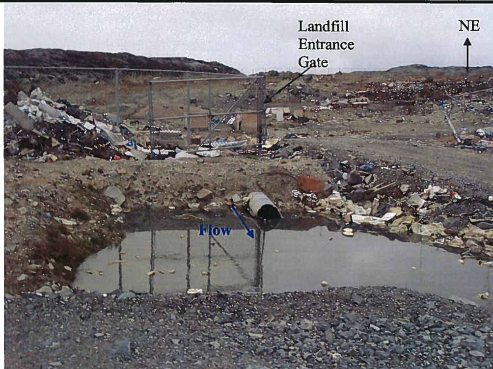
Photo 7: Entrance to landfill area, culvert draining water out of landfill
