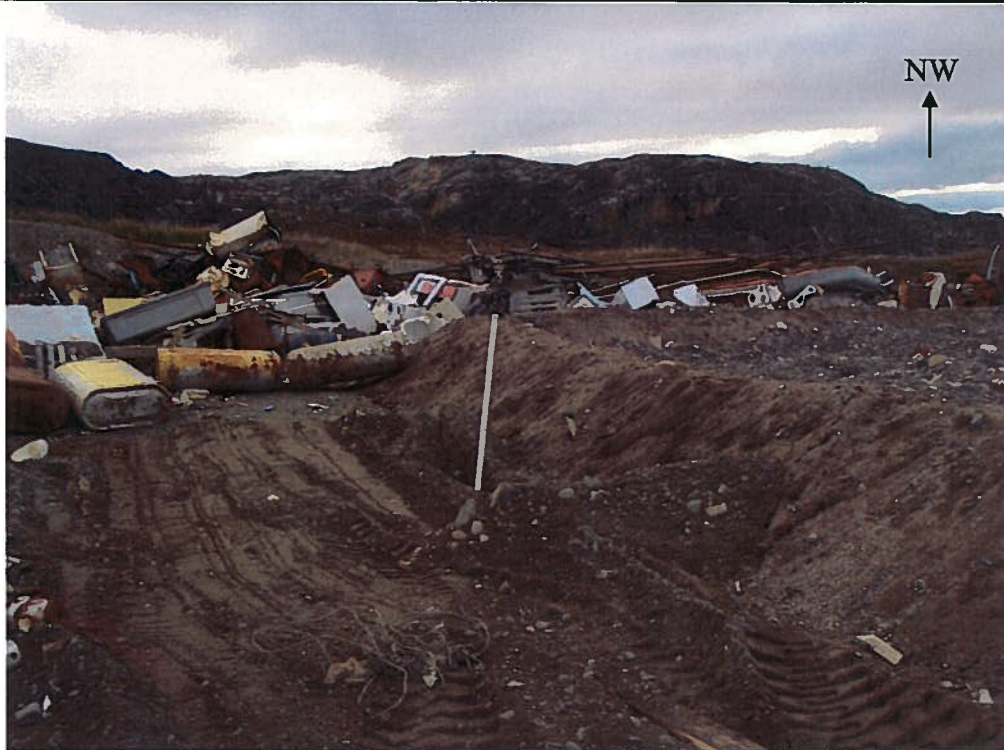
Photo 20: Monitoring well installed at landfarm
