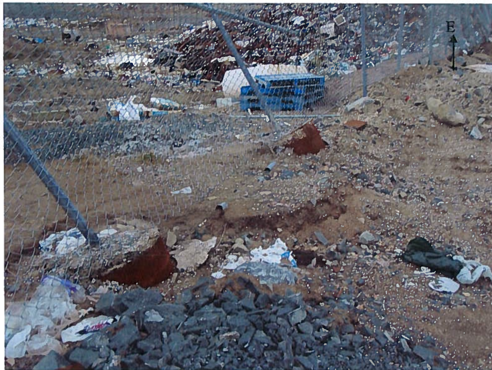
Photo 6: Barrels in ground securing fence posts heaved out of ground. Looking east.
