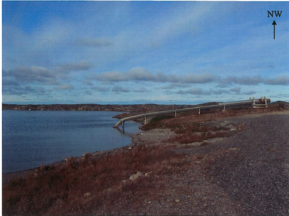
Photo 13: Sewage Lagoon flute pipe where trucks discharge sewage into lagoon.
