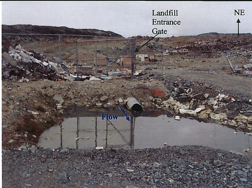
Photo 3: Entrance to landfill area, culvert draining water out of landfill
