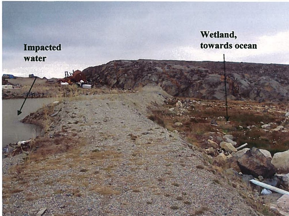
Photo 7: Berm holding water from landfill from discharging to ocean. Looking SW.
