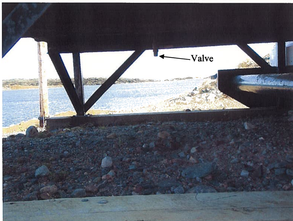
Photo 8: Valve to empty water from containment around fuel storage tank
