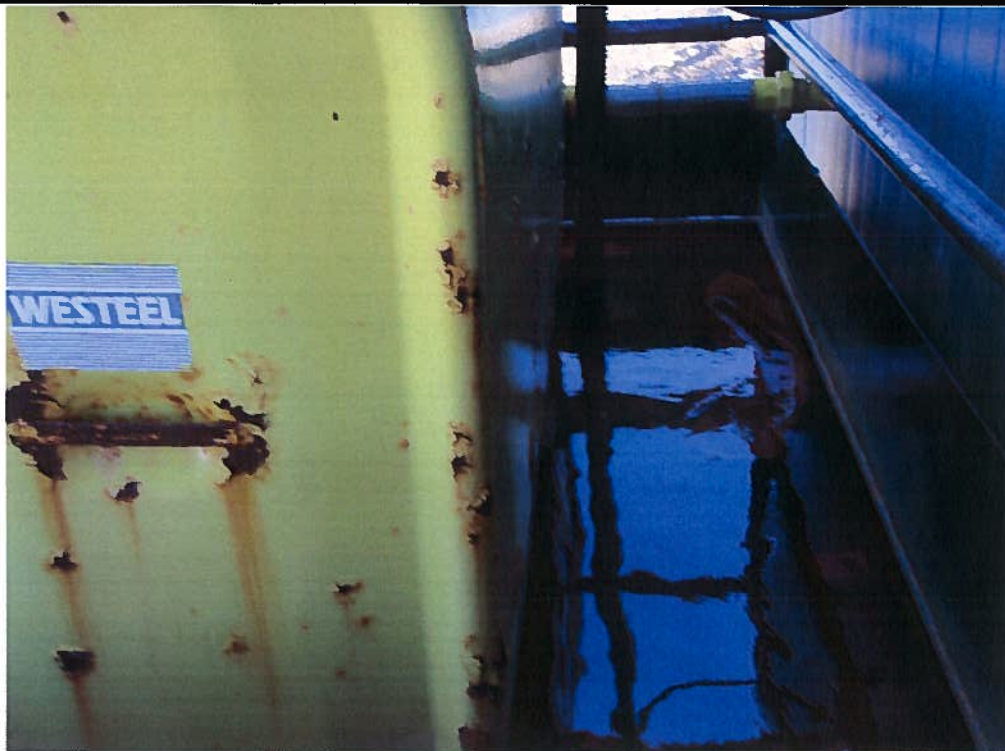
Photo 7: Water around pump house fuel storage tank
