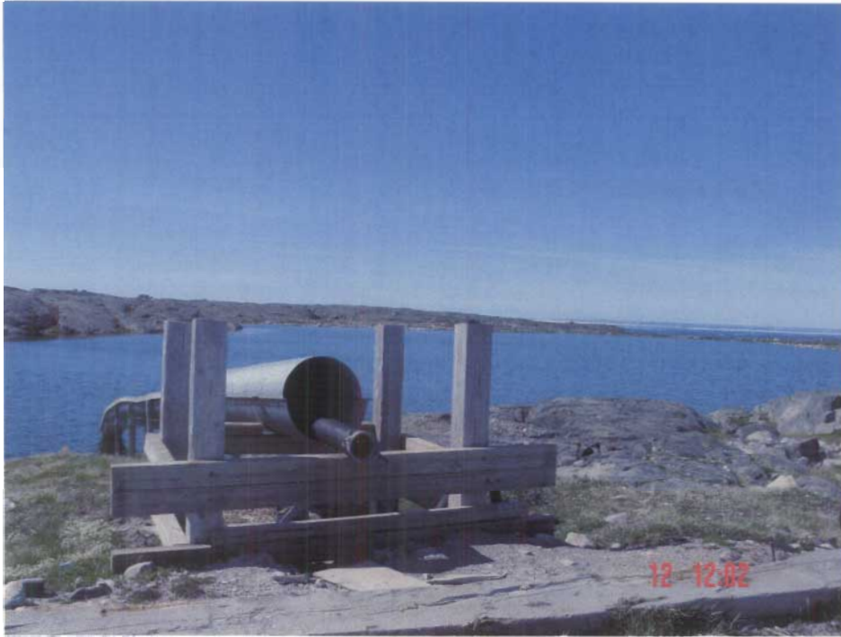
Photo # 5 Sewage truck discharge structure at Sewage Treatment Facility.
