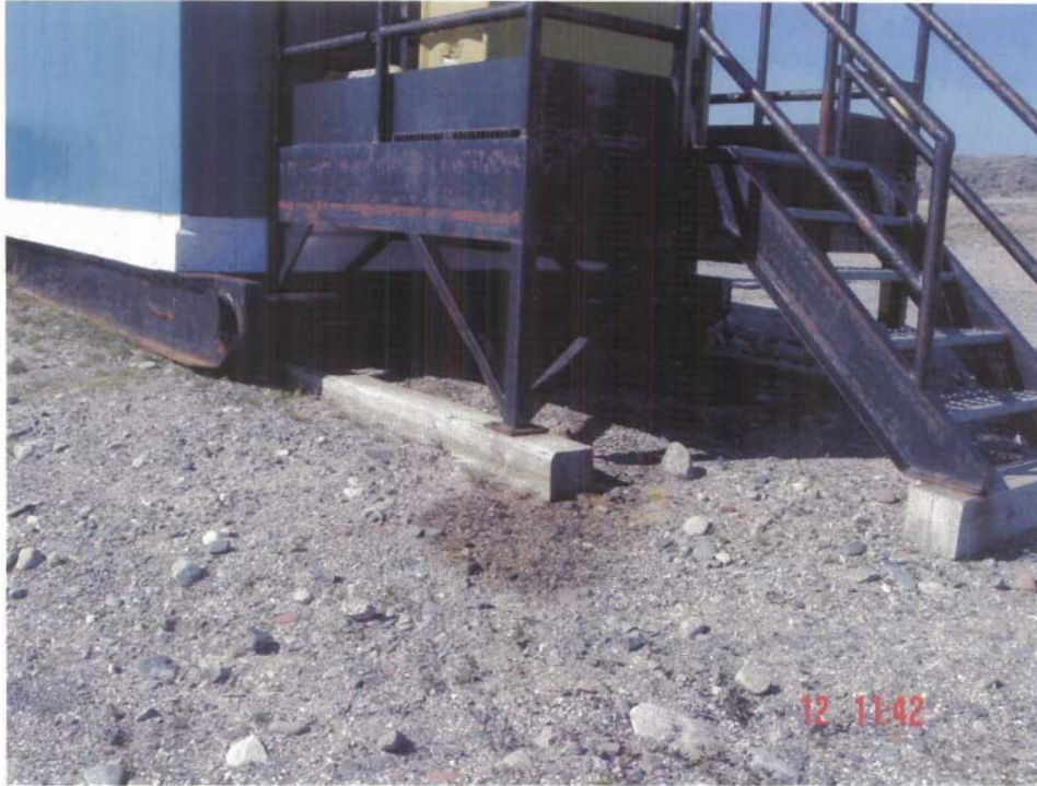
Photo # 3 Spilled fuel oil was noted at the time of inspection. No spill protection or recovery equipment was available at the intake facility.
