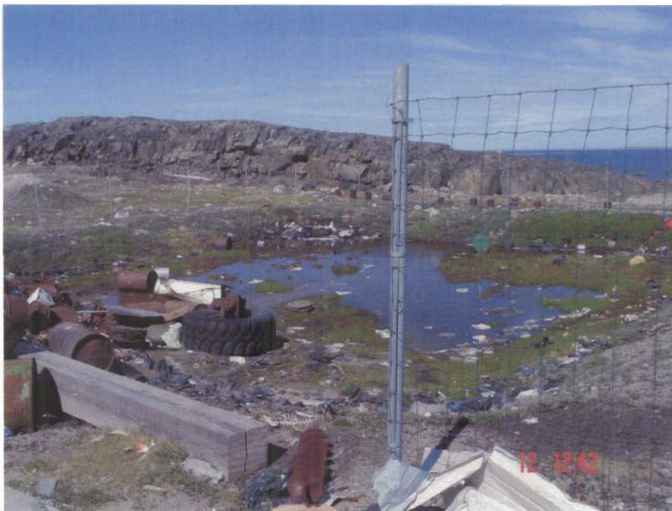
Photo # 8 Old sewage lagoon shown in solid waste disposal grounds. Liquid noted in picture was seen leaching out into ocean.
