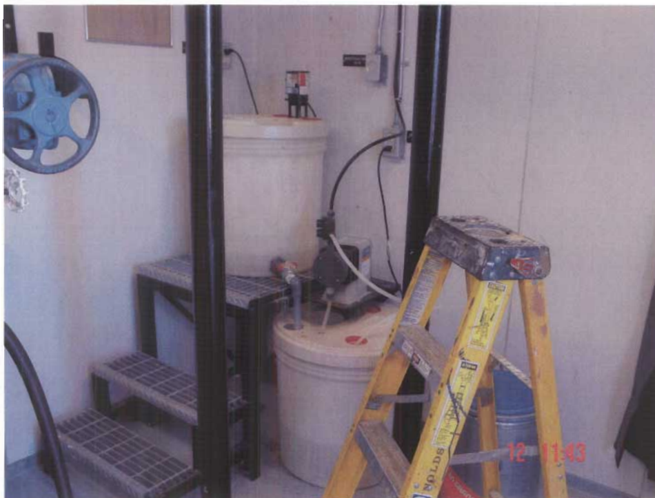
Photo # 3 Spilled fuel oil was noted at the time of inspection. No spill protection or recovery equipment was available at the intake facility.
