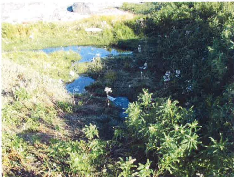
Photograph No. 16: Minor Berm Seepage (West Berm)
