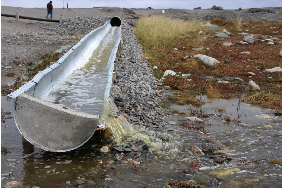
Figure 11 Discharge dispersion structure close up
