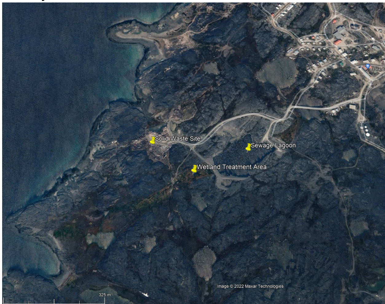
Figure 1 Whale Cove Sewage Disposal Facility
