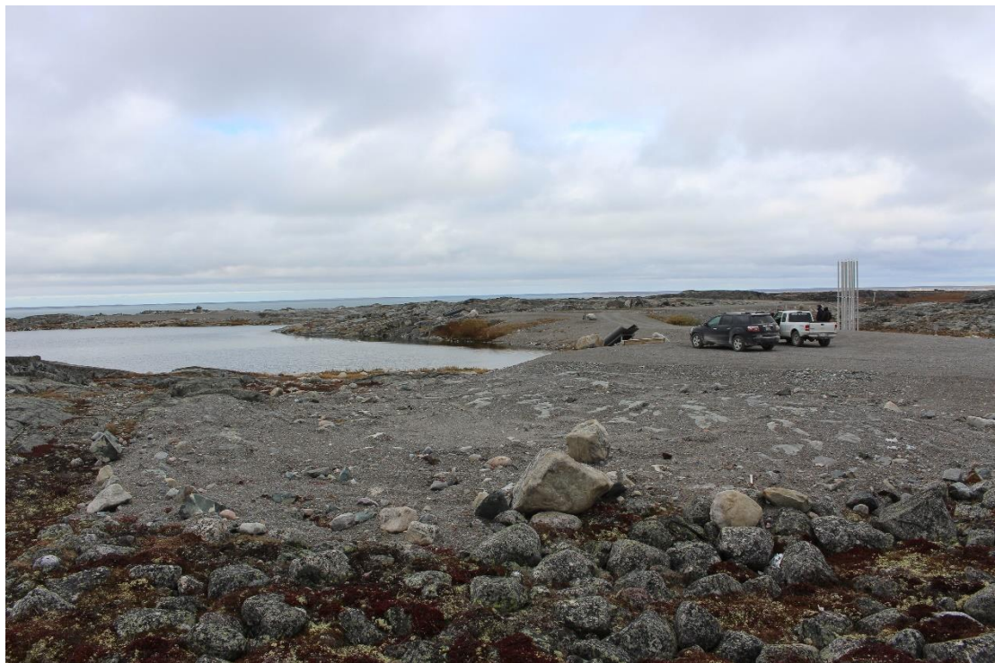
Figure 6 Northeast lagoon berm
