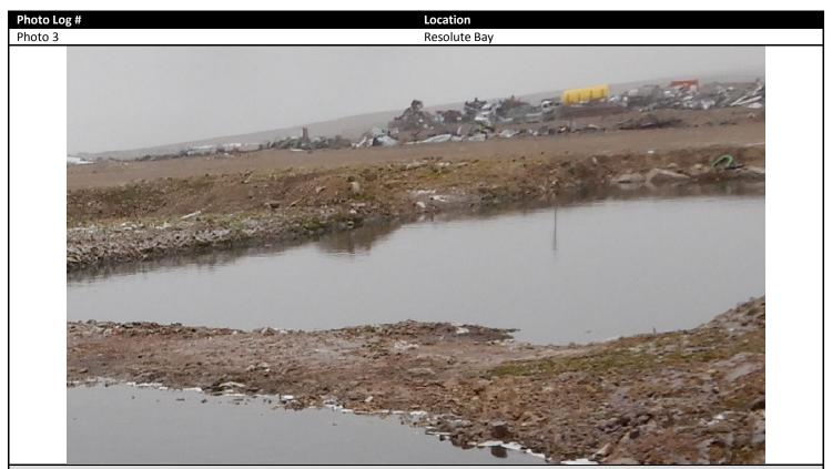
Description: Walls on the north side shows less than 1 metre freeboard. The sludge on the ground shows the height of walls of Sewage Disposal Facility
