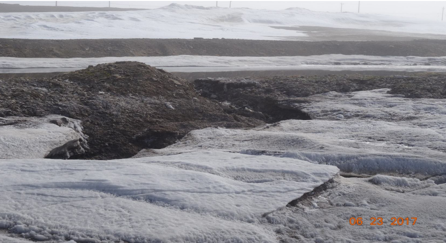
Figure 2: Erosion of cell #1 leading to cell #2
