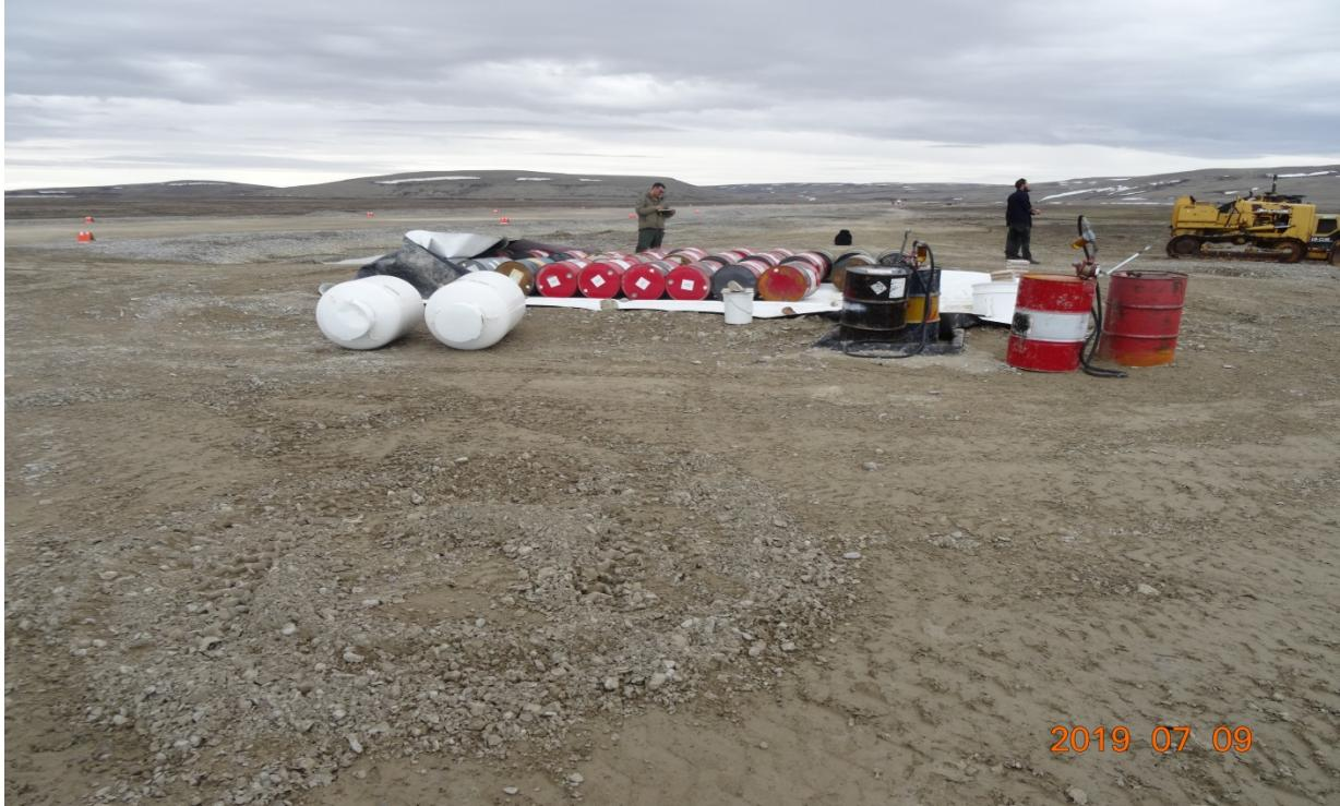
**Description:** Fuel Cache secondary containment walls are flush with the surrounding landscape. 19 barrels on top of liner. Also a fuel transfer station.
