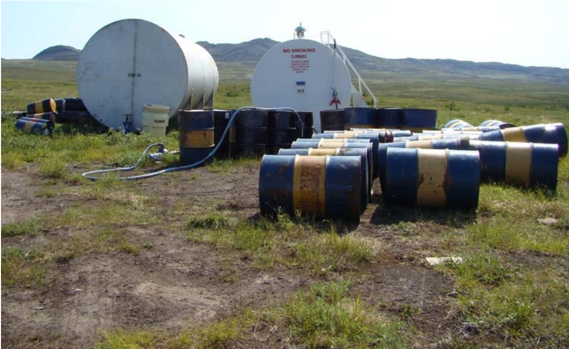
Photograph 22: Area used for re-filling fuel drums. No secondary containment is used: pump is directly on ground and fuel nozzle is left to drip on the ground. Note darker staining of soil in lower right foreground.
