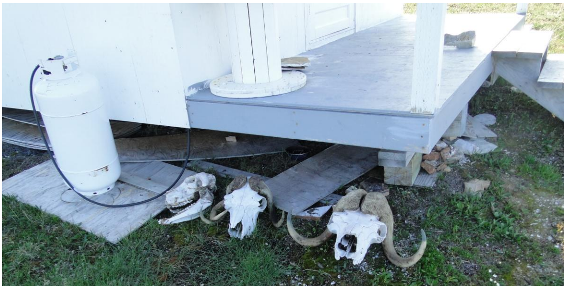
Figure 2. Tall propane tank, not fixed to building.
