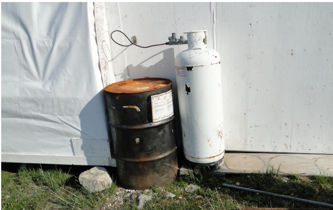
Figure 4. Fuel drum, not in containment.
