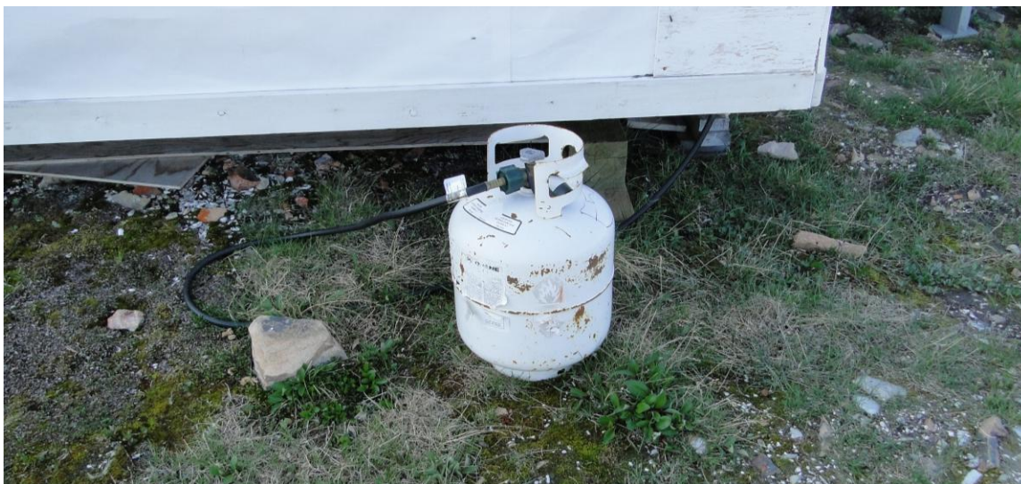
Figure 3. Small propane tank, not fixed to building.
