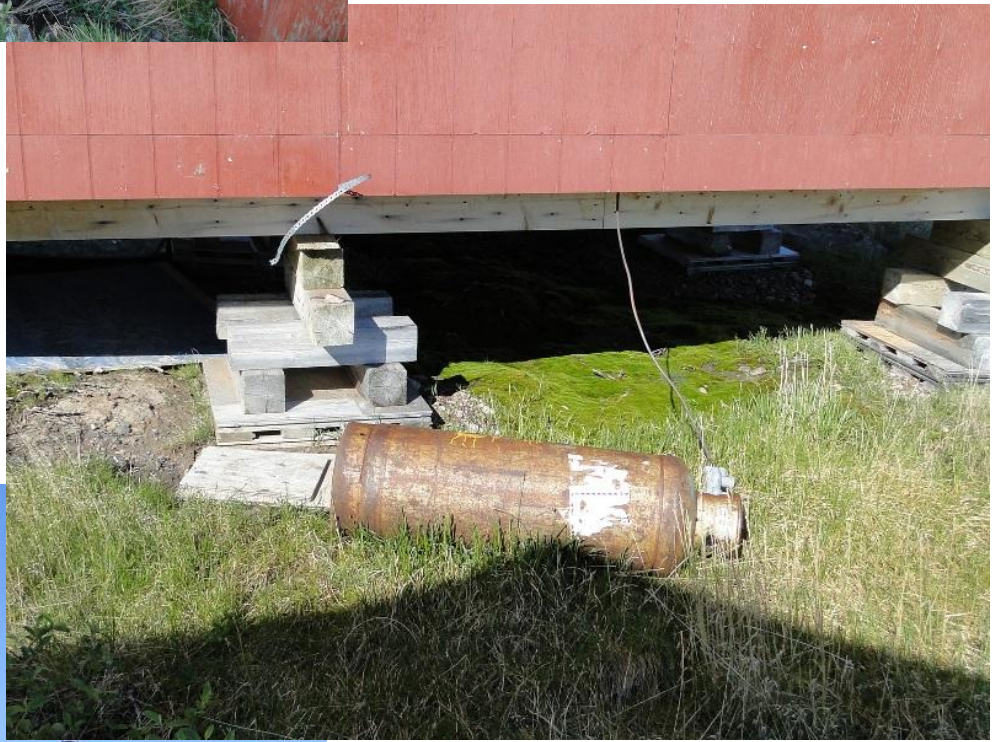
Figure 7. Propane tank has come loose.
