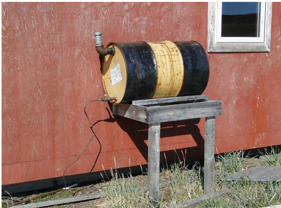
Figure 5. All fuel barrels should be over a berm.
