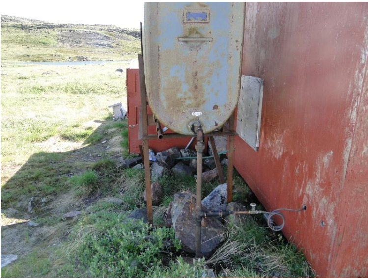
Figure 6. Containment under valve and hose required.
