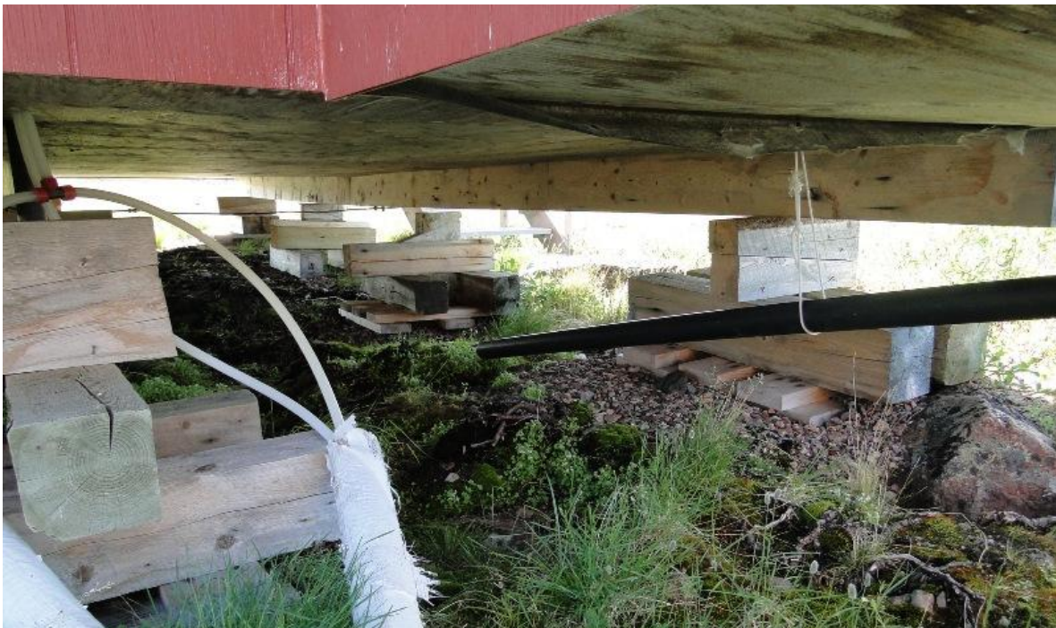
Figure 2. Water discharge directly under each cabin.
