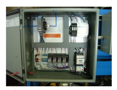
Control panel for Moyno pump (detail)
