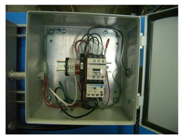
Control panel for Gould's pump (detail)
