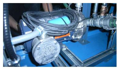
Gould's Centrifugal Transfer Pump
