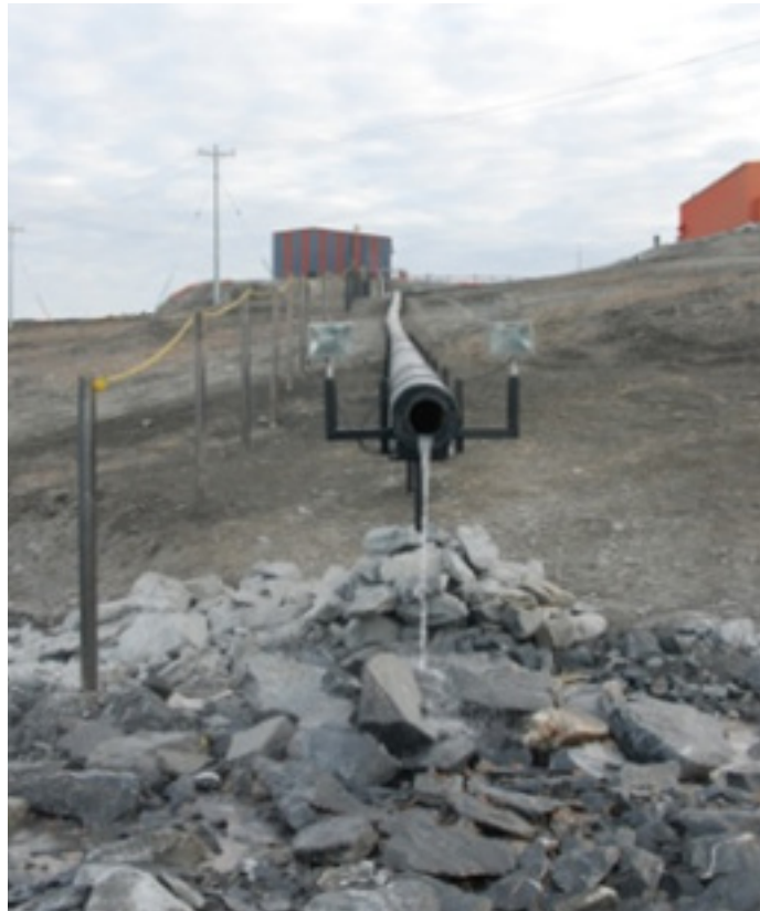
Figure 1.2. The discharge pipe delivering wastewater to the wetland
